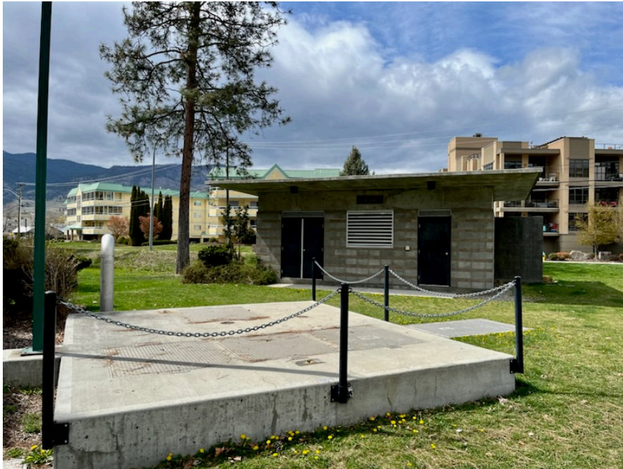
Figure 2 –Lee Ave. Lift Station
