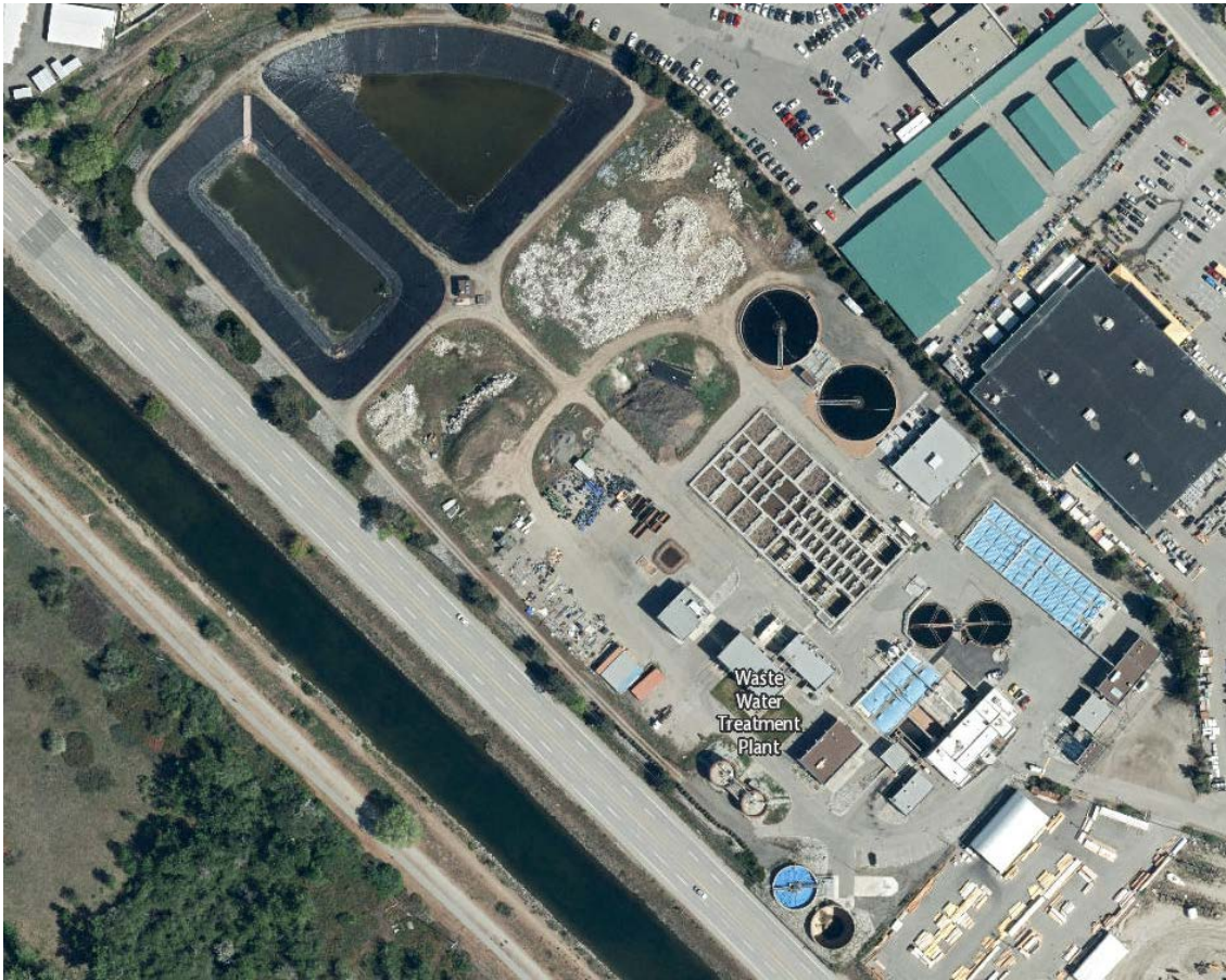
Figure 1 – Aerial View of AWWTP
