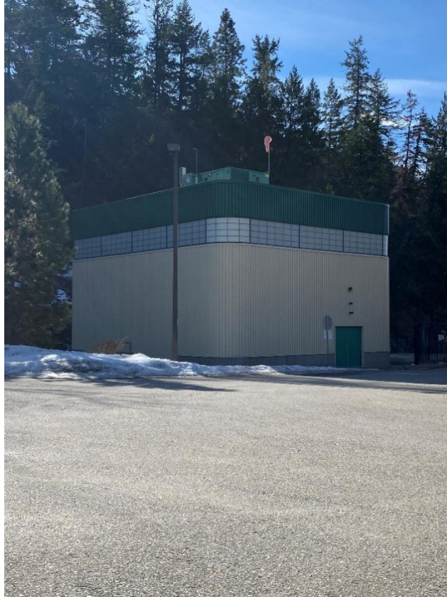
Figure 12. Penticton Water Treatment Residual Handling Building
