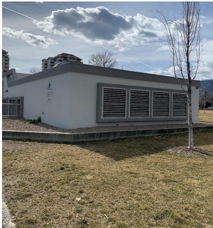
Figure 5. Okanagan Lake Pump Station
