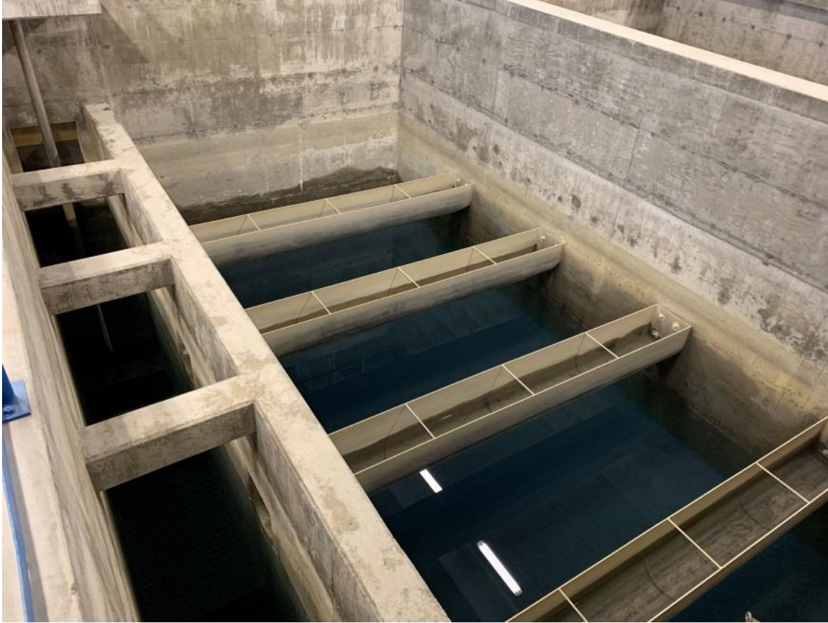
Figure 11. Penticton Water Treatment Mono Media Filters
