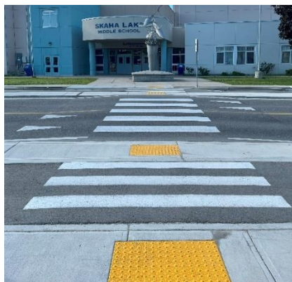
Main Entrance Raised Crosswalk
