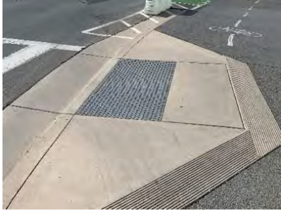
Example of accessible curb ramp
