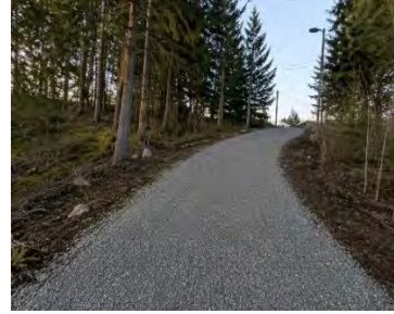
Compacted aggregate trail
