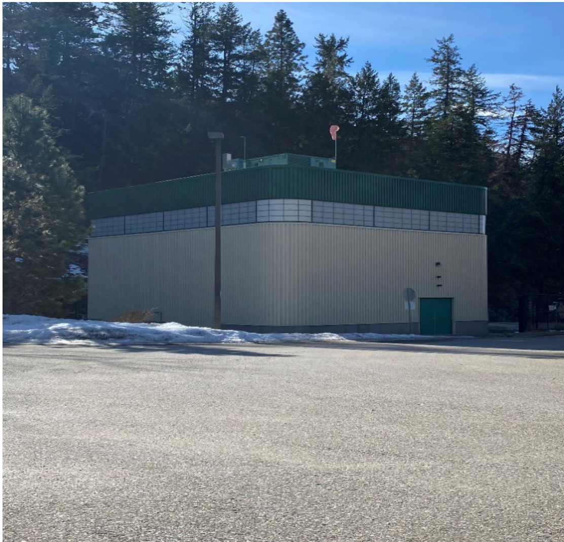
Figure 11. Penticton Water Treatment Residual Handling Building
