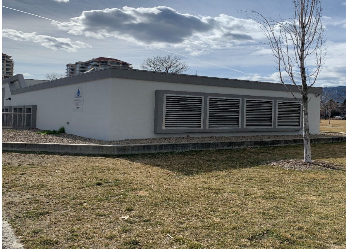
Figure 5. Okanagan Lake Pump Station
