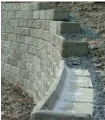
Example of "mass" retaining wall
