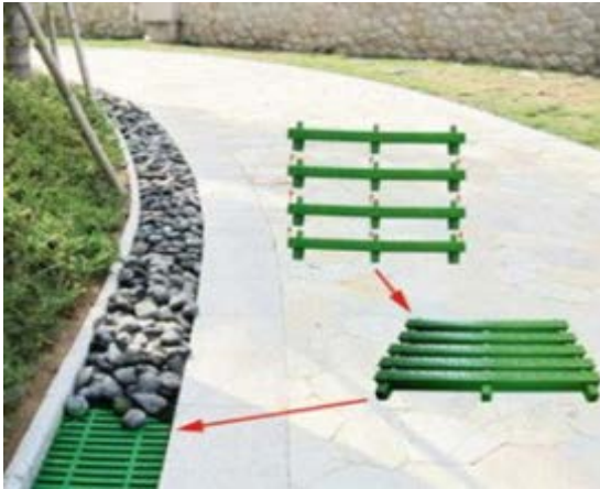
On-site Drainage Control
