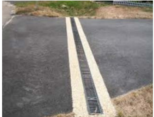
Driveway to Boulevard trench
