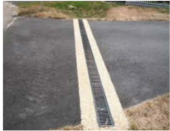
Driveway to Boulevard Trench
