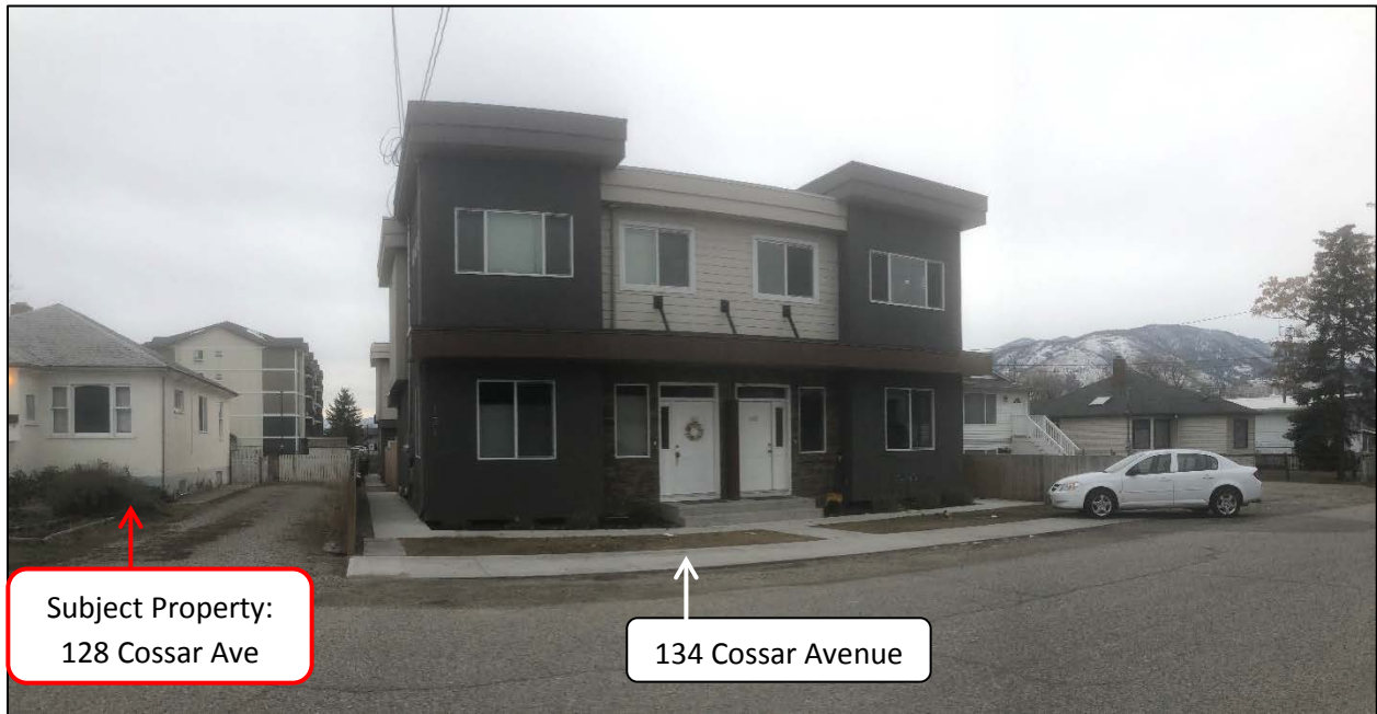
Looking down western property line from Cossar Avenue (next to 134 Cossar Avenue development)
