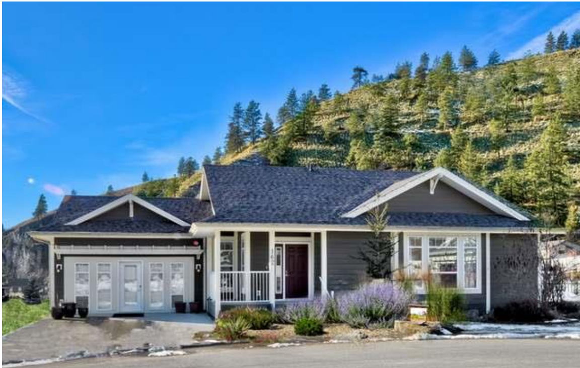
Figure 35: Single family home on Penticton Ave
