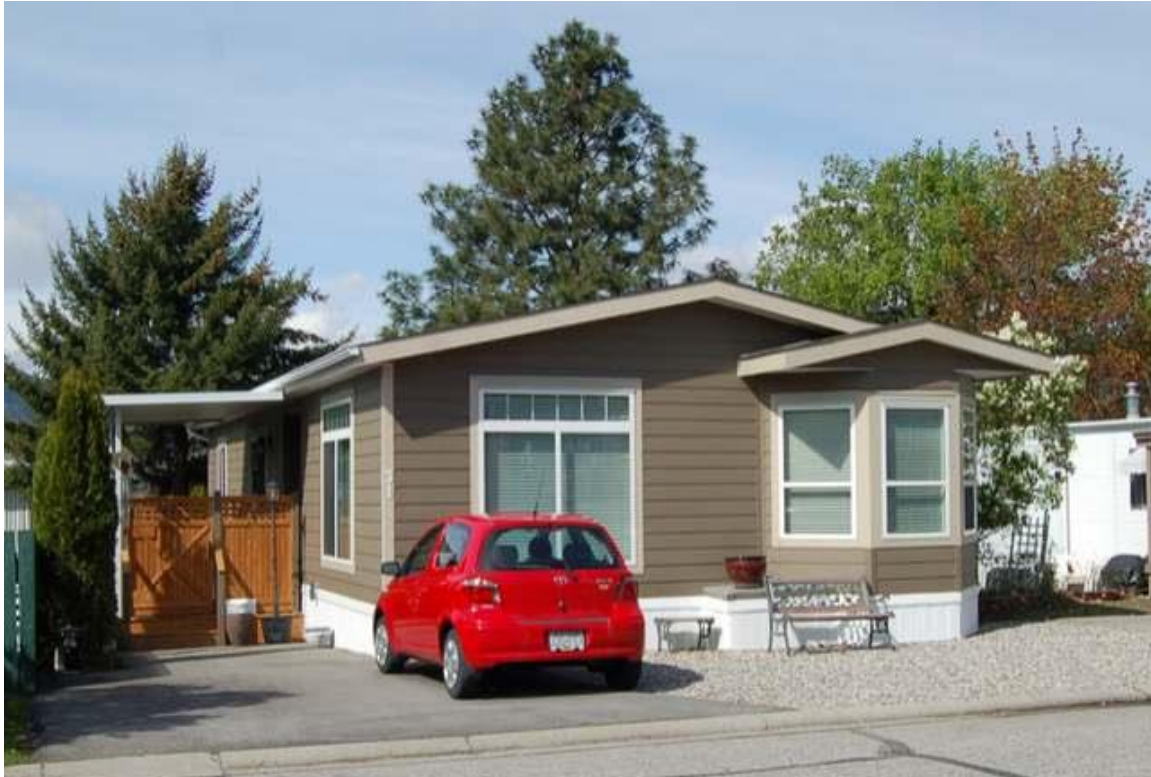
Figure 44: Mobile home: 31-98 Okanagan Ave E
