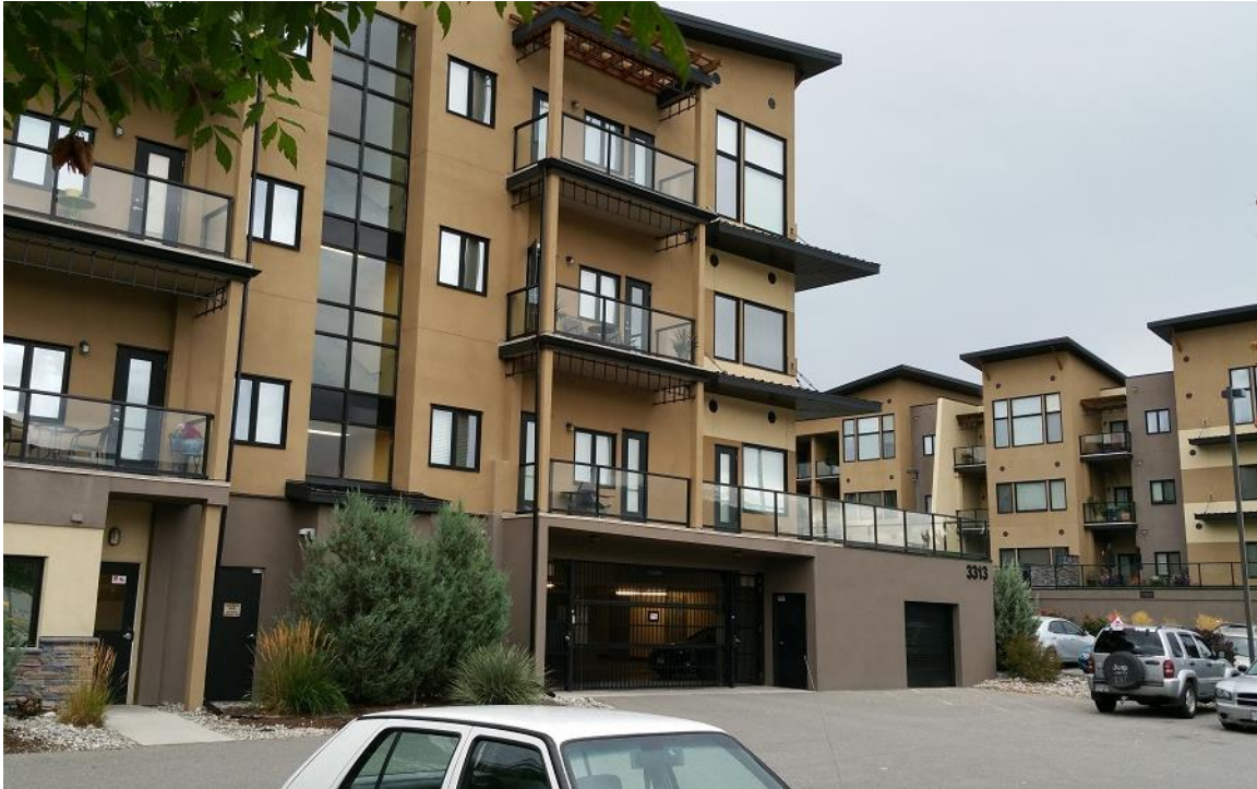
Figure 42: Three storey condominium over podium
