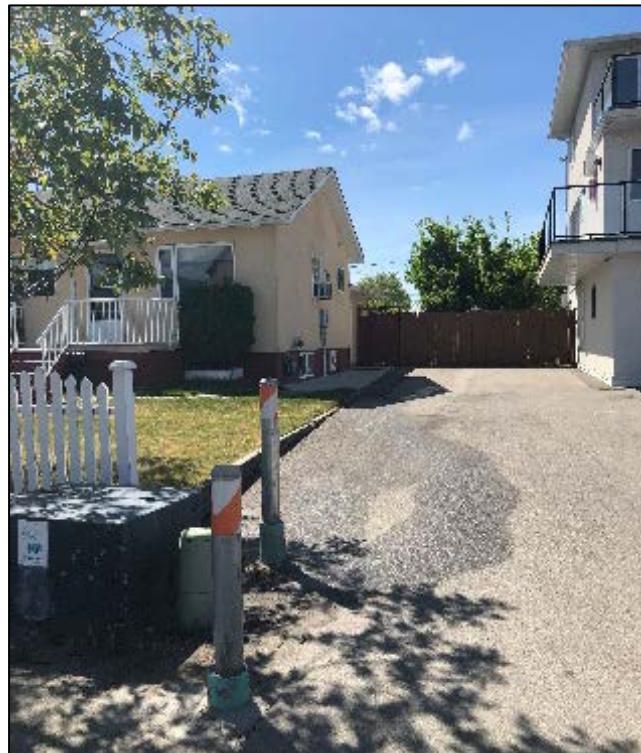
Figure 8 – Looking down eastern property line of 1050 Churchill Avenue
