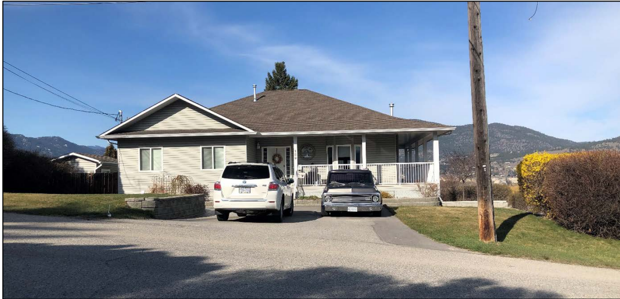
Looking towards front of house from Grandview Street
