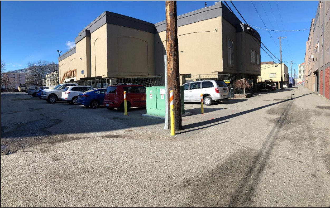
Looking north towards existing building from laneway
