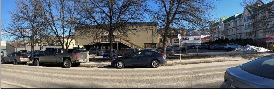
Frontage of Property (west elevation)
