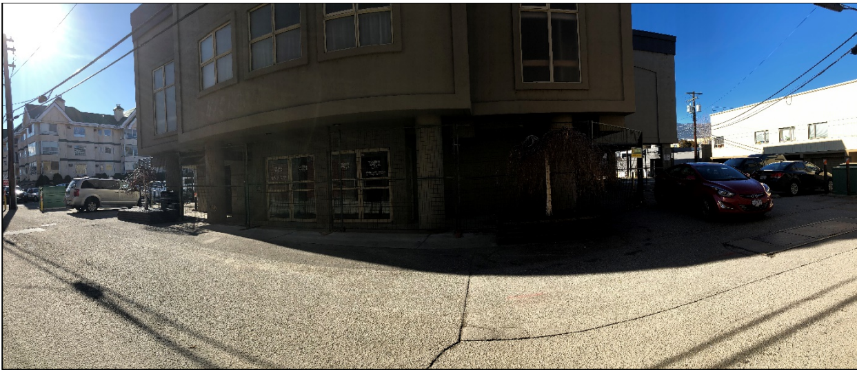
Rear of Existing Building (looking west)
