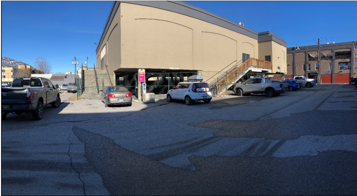
South Elevation of Existing Building
