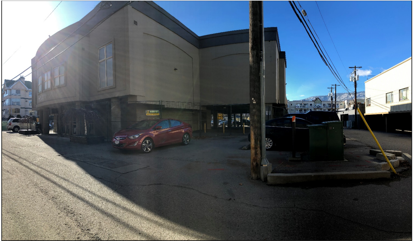
Looking West at Northeast Corner of Property
