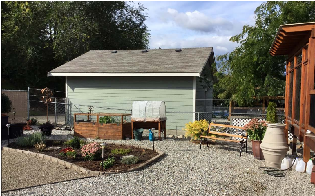
View of existing garage from (east) neighbouring property
