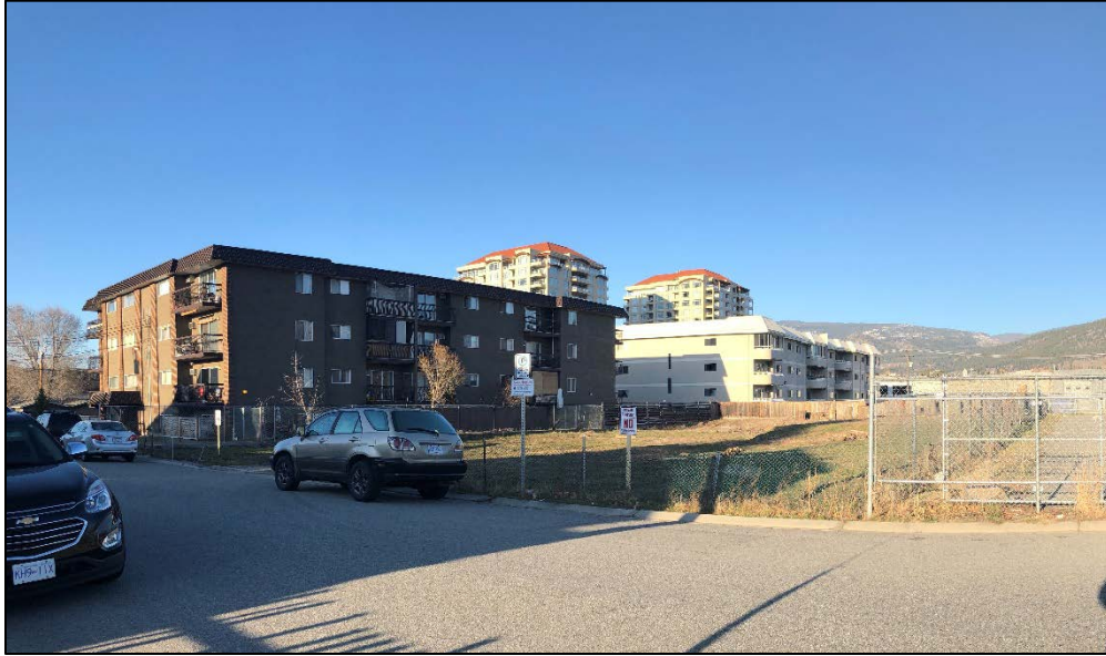
Looking towards subject property from Brunswick Street
