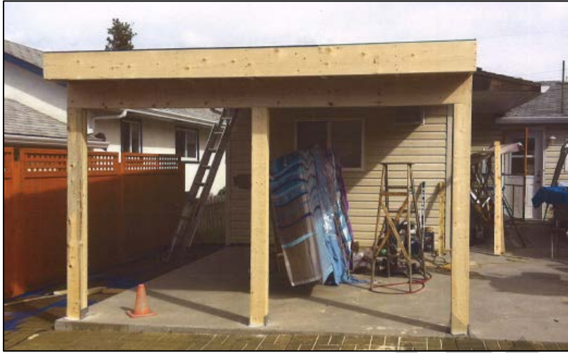
Figure 2 - Image of covered patio addition, proposed to be enclosed.
