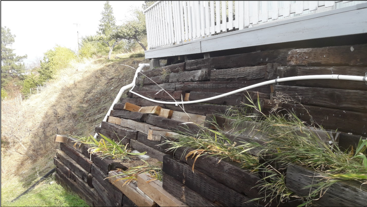
Photo of original wood retaining wall
