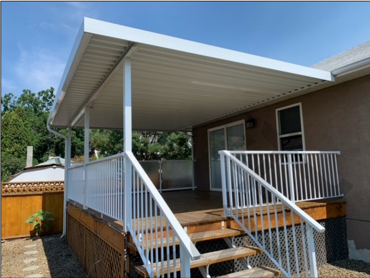
Existing deck to be legalized
