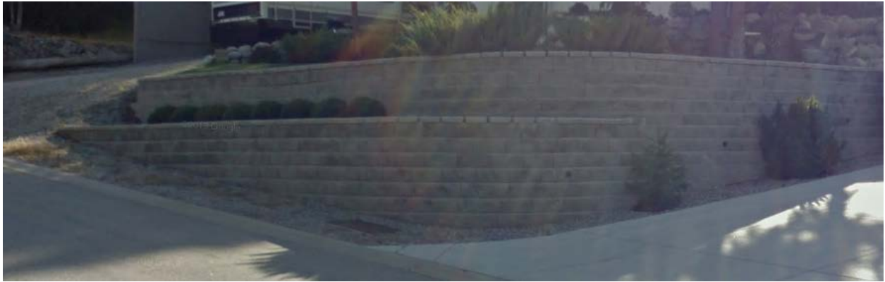
Figure 3 - Example retaining wall across Evergreen Dr from subject property
