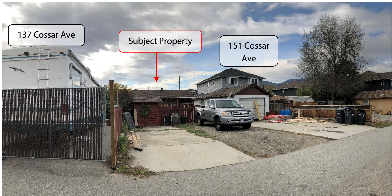
Looking towards subject property from laneway
