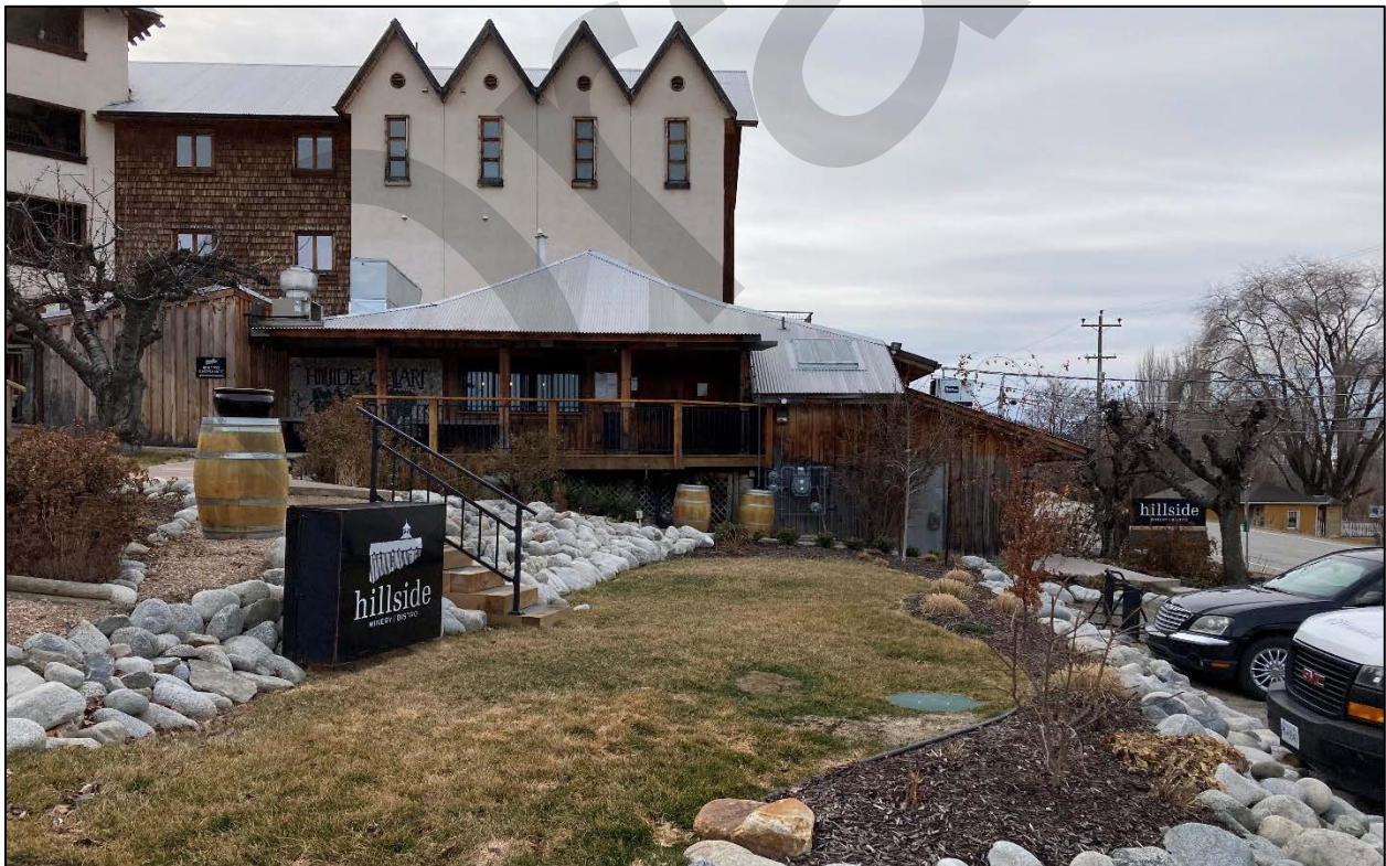
Looking towards area of outdoor lounge expansion
