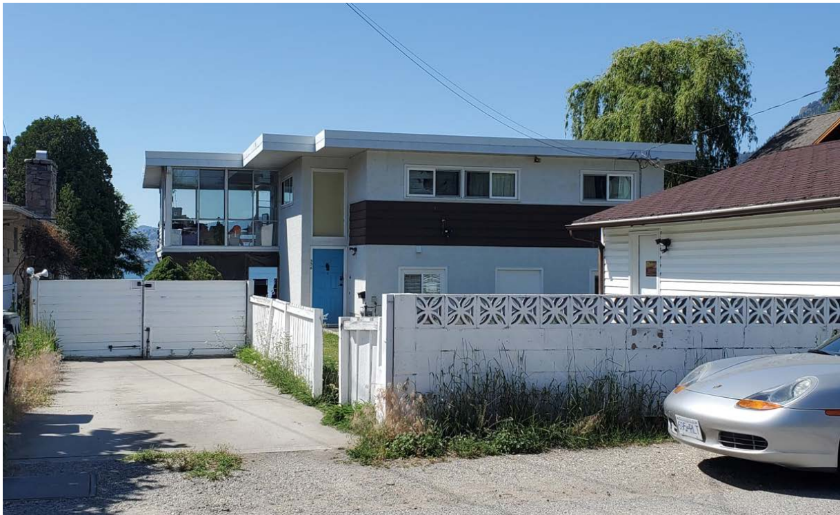
Figure 4: View of the house towards Skaha Lake
