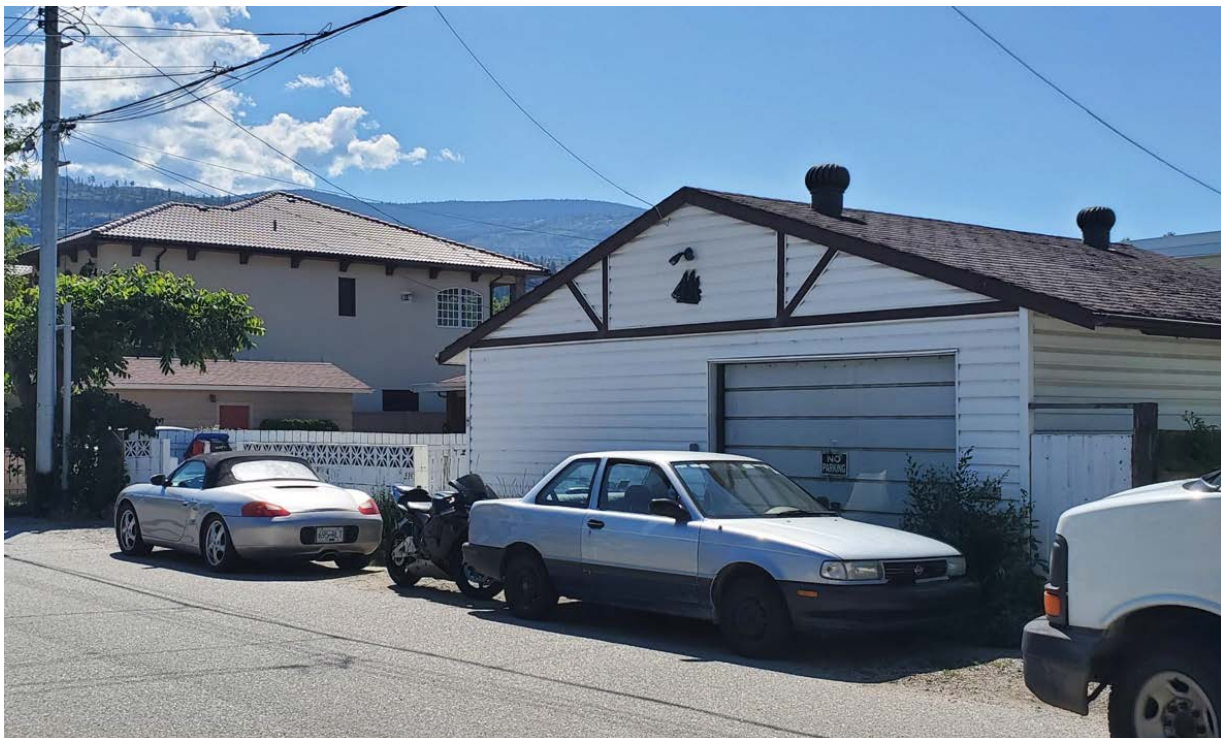
Figure 5: View of existing garage looking north
