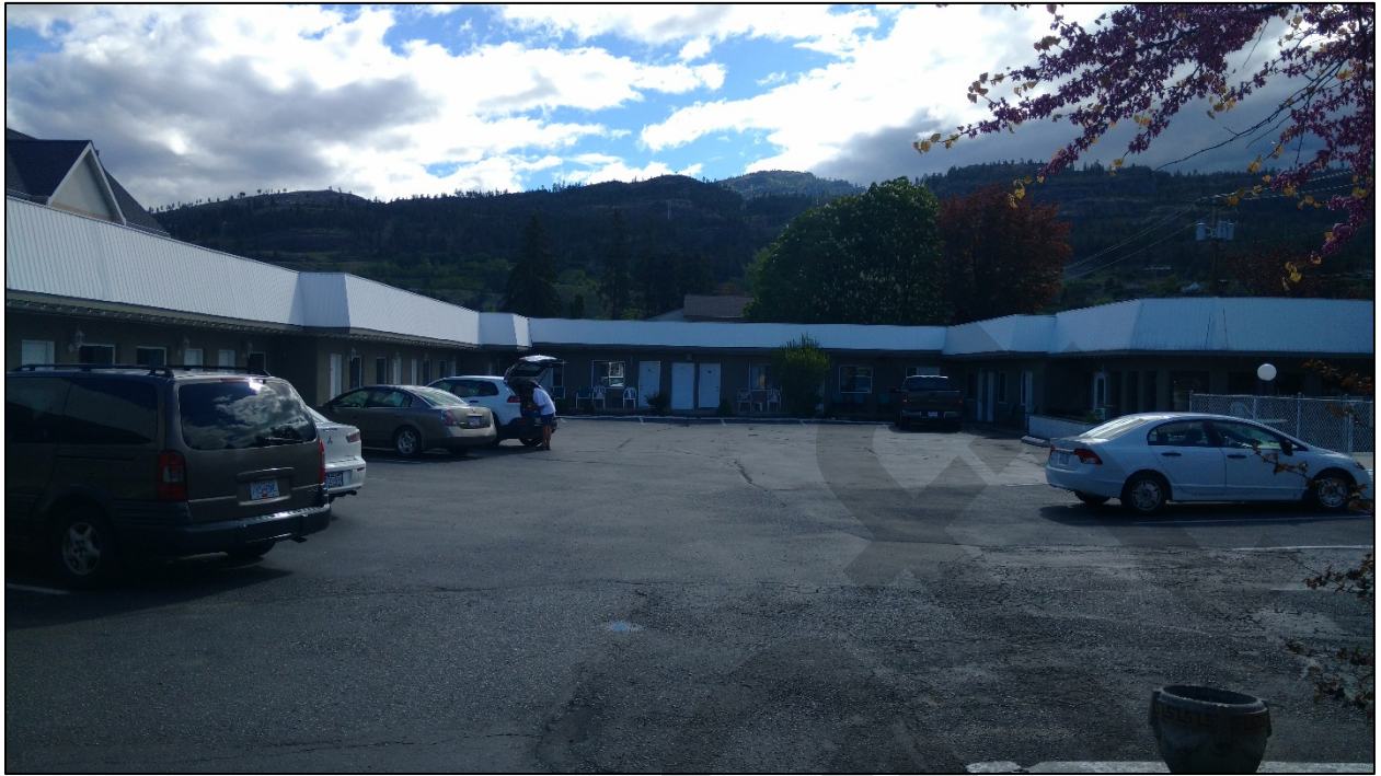
Figure 10: Existing motel parking lot
