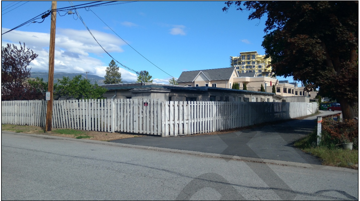
Figure 8: South East view of property
