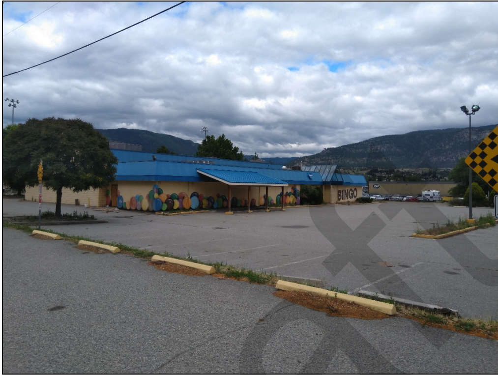
Figure 6: North East View (from the lane)
