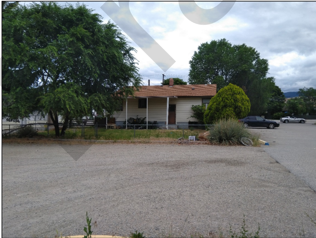
Figure 11: South View showing back of existing dwelling
