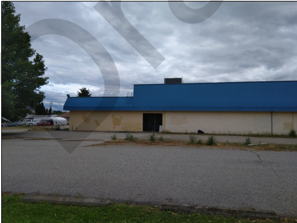
Figure 9: South View showing back of existing Bingo Hall
