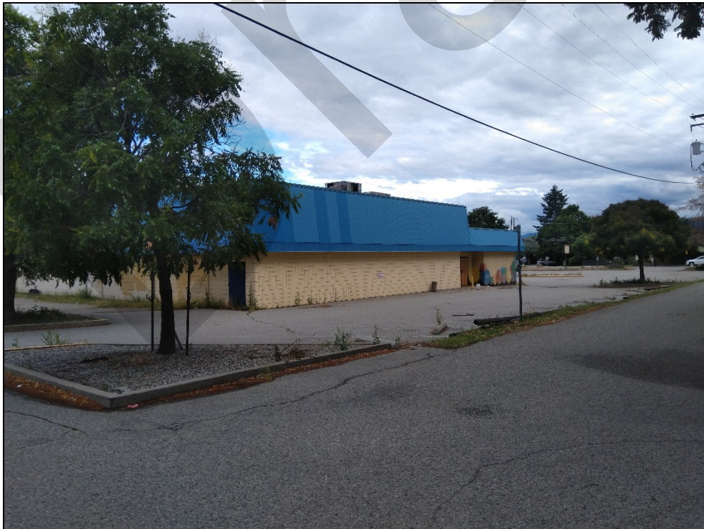
Figure 7: South East View (from the lane)
