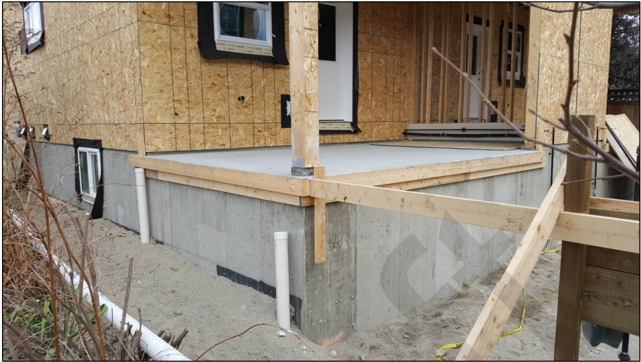
Figure 6 – Looking at the deck of one of the units (over 0.6m from finished grade)
