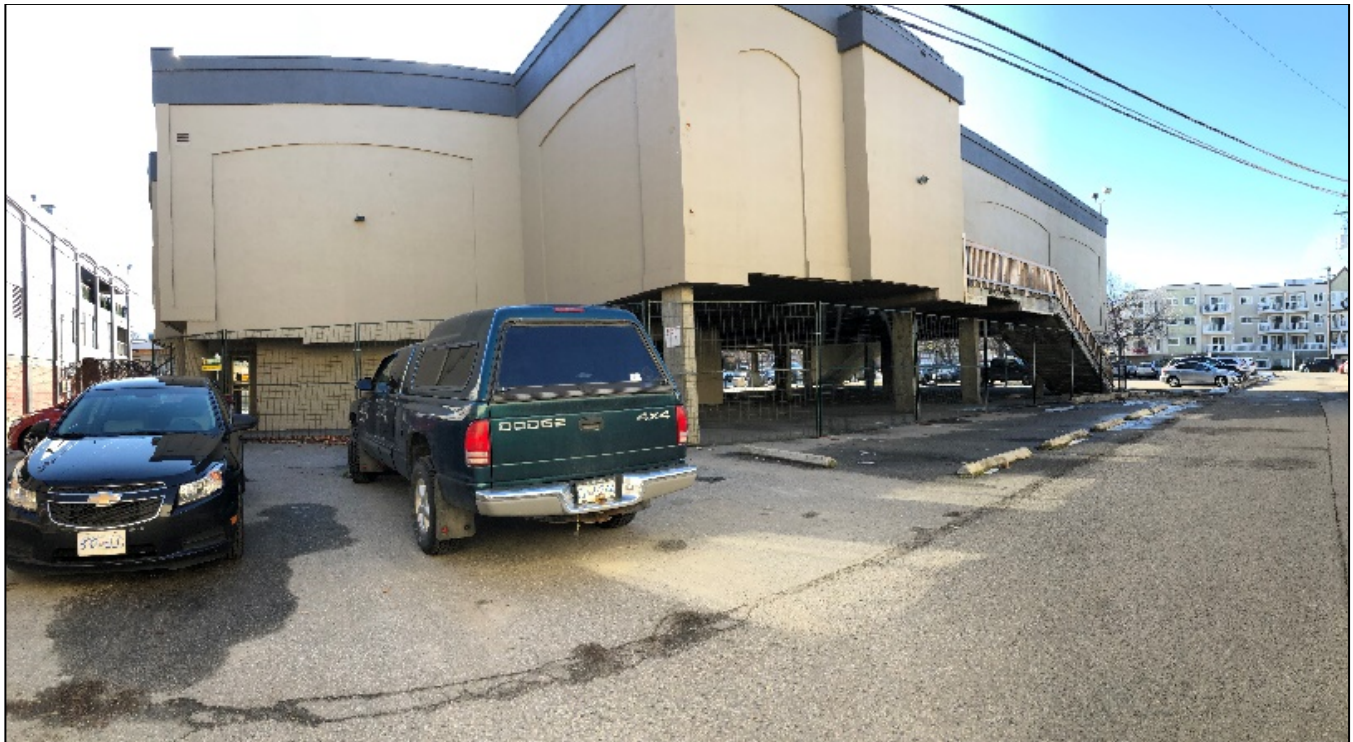
Looking South at North Elevation of Existing Building from laneway
