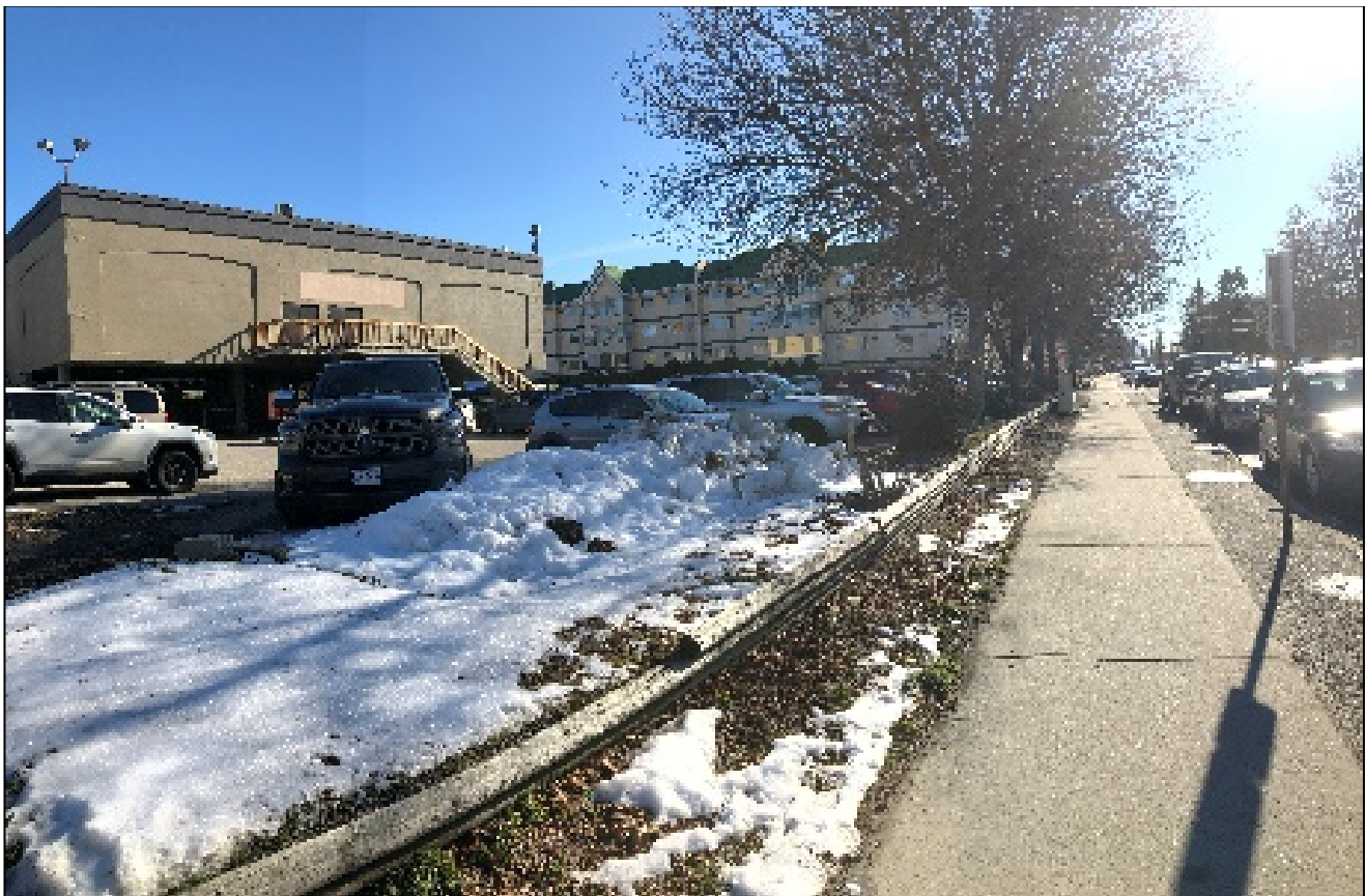
Looking south along existing property frontage
