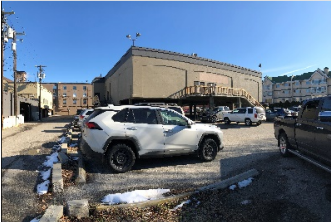
Looking east from northwest corner of property
