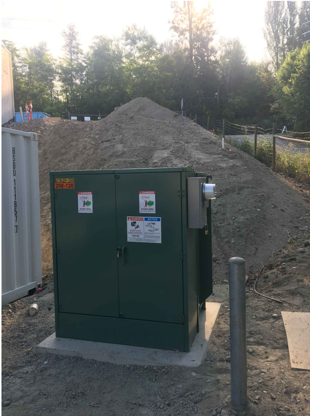
Pad Mount Transformer Metering
