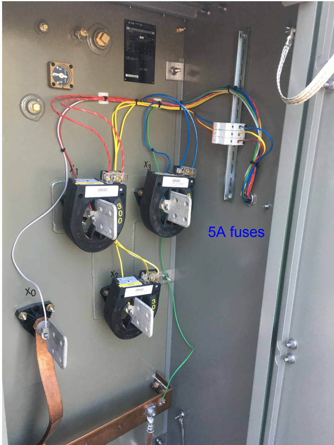
Pad Mount Transformer Metering
