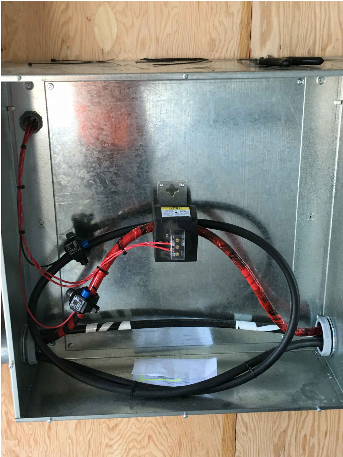
5 Jaw SC Meter Connections 1 Phase 120/240V Y
