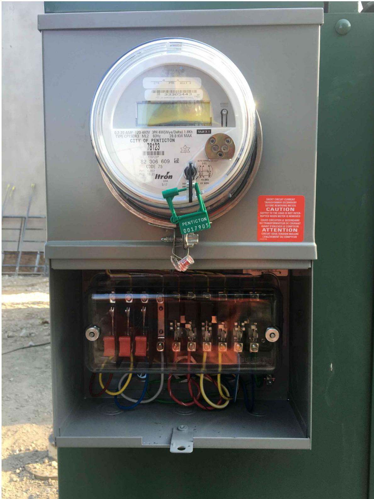
13 Jaw SC Meter Connections 3 Phase 120/208\text{V} Y & 347/600\text{V} Y
