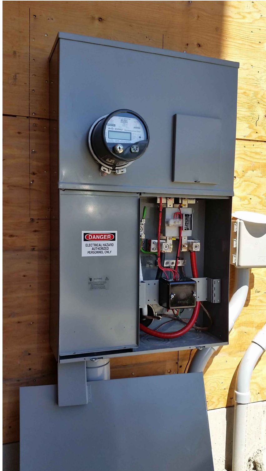
Single Phase Residential Service 400A 120/240V All in One Transformer Rated Meter Socket
