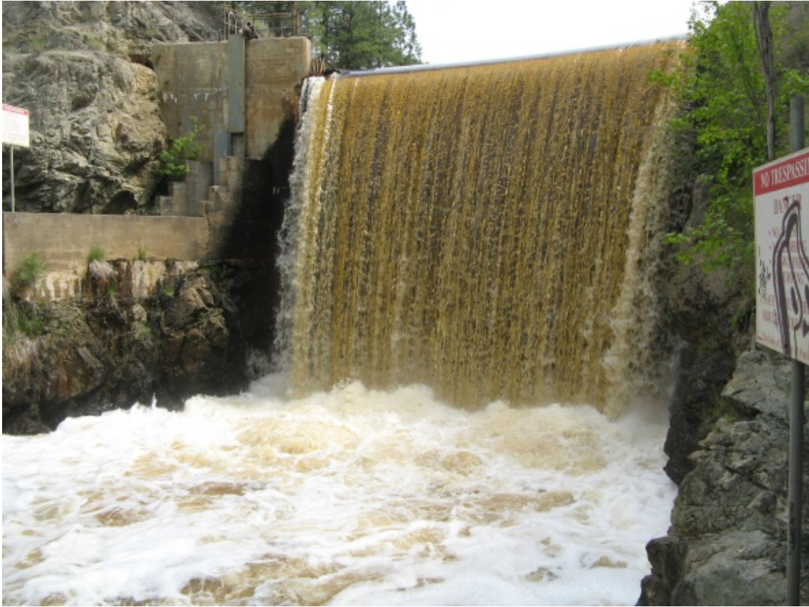
Figure 1: Penticton Creek Dam 2
