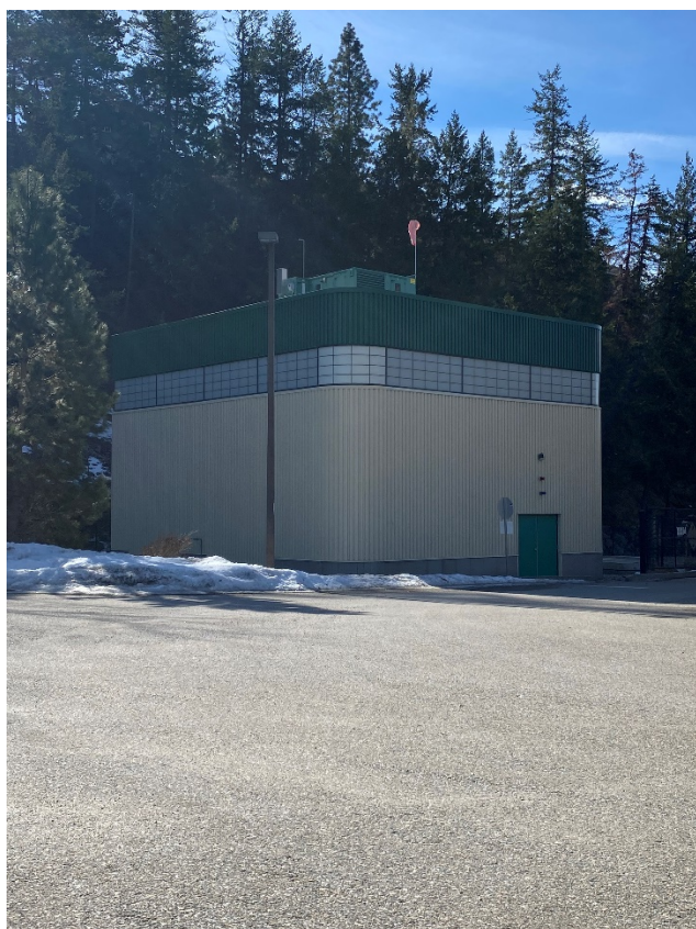
Figure 12: Penticton Water Treatment Residual Handling Building
