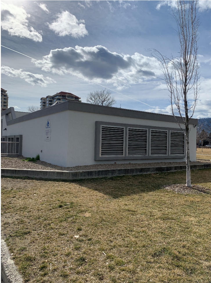
Figure 5: Okanagan Lake Pump Station
