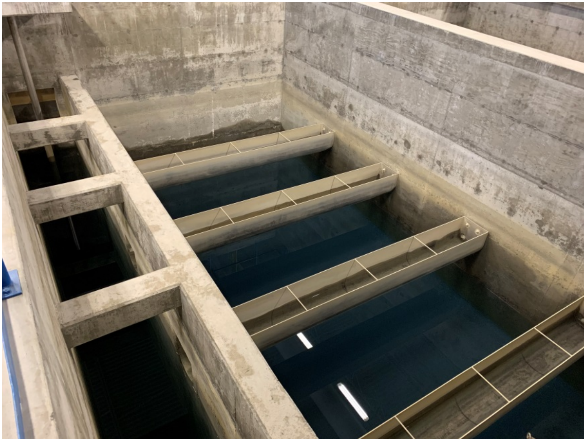
Figure 11: Penticton Water Treatment Mono Media Filters
