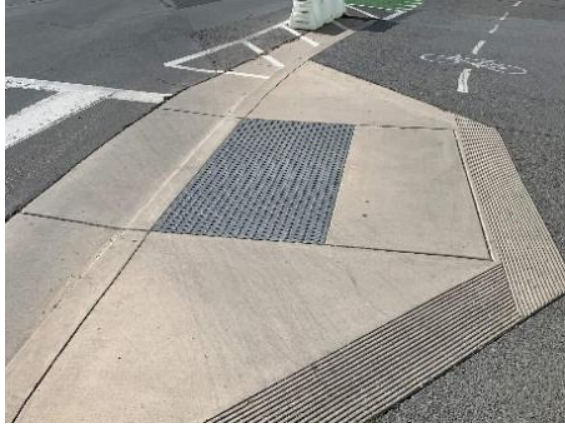
Example of accessible curb ramp
