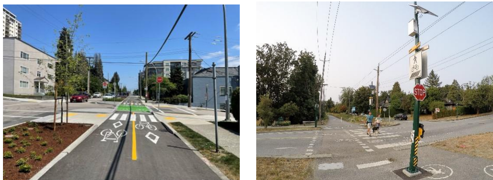
Examples of protected intersection crossing improvements with curb extensions and RRFBs
