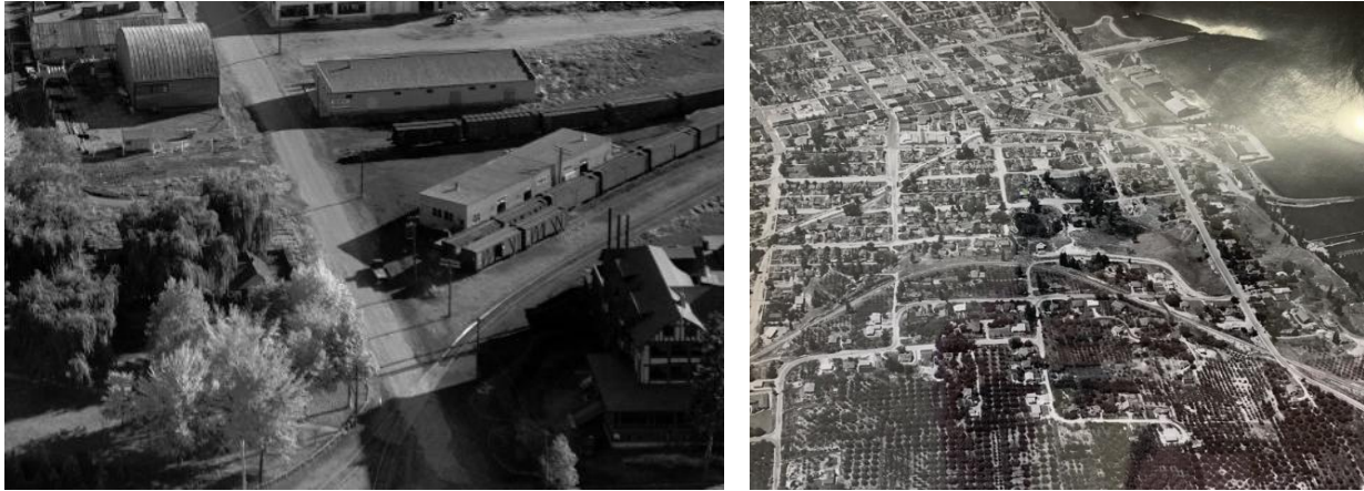
Historical photos showing the original KVR corridor through the City of Penticton (Source: City of Penticton)
