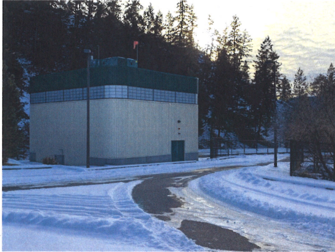
Figure 9: Residual Handling Building
