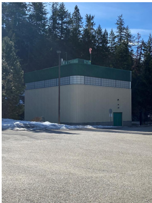
Figure 13: Penticton Water Treatment Residual Handling Building
