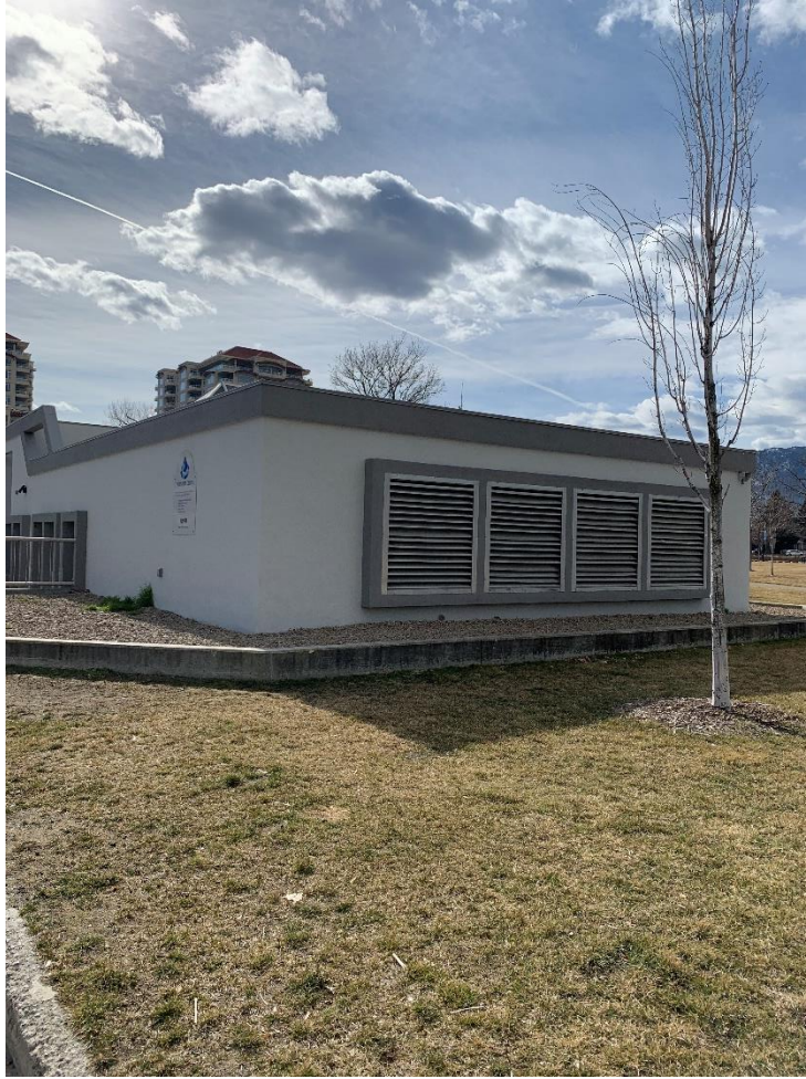
Figure 6: Okanagan Lake Pump Station
