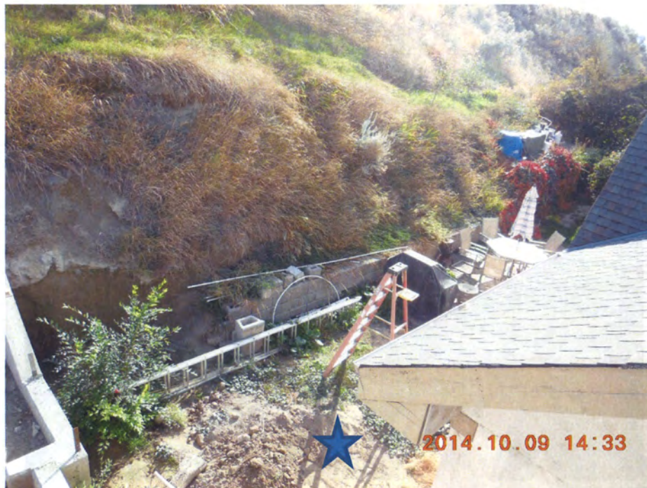
Drainage work taking place
