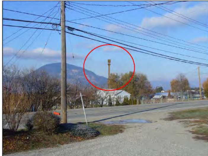
Looking Northwest from Upper Bench Road South
