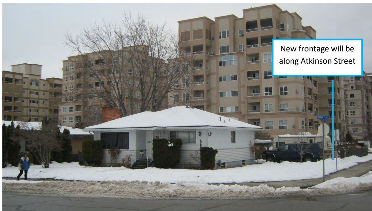
Figure 4: Front of 115 Kinney Avenue with Cherry Lane Towers in background
