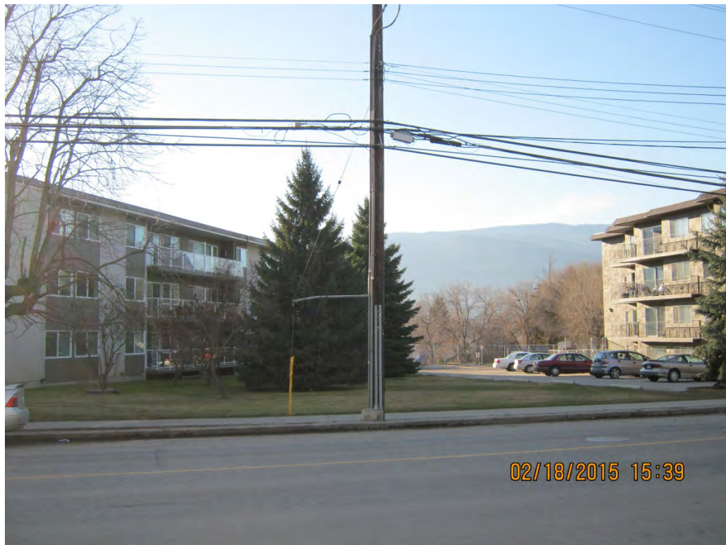
Figure 5: Looking west at 783 Winnipeg St. from across Winnipeg St.
