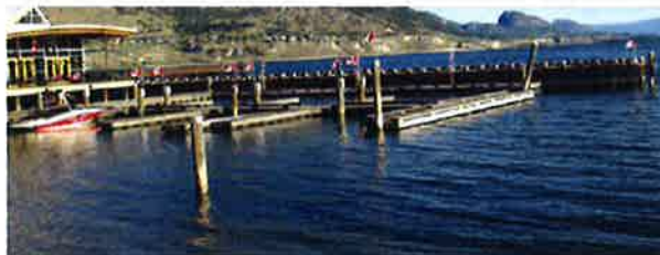
Fig. 5. View of dock at Penticton Lakeside Resort.
