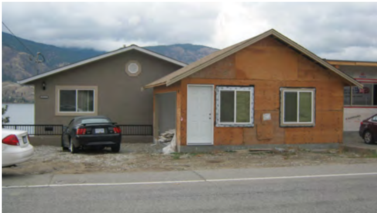
Figure 3: Looking west at front face of building
