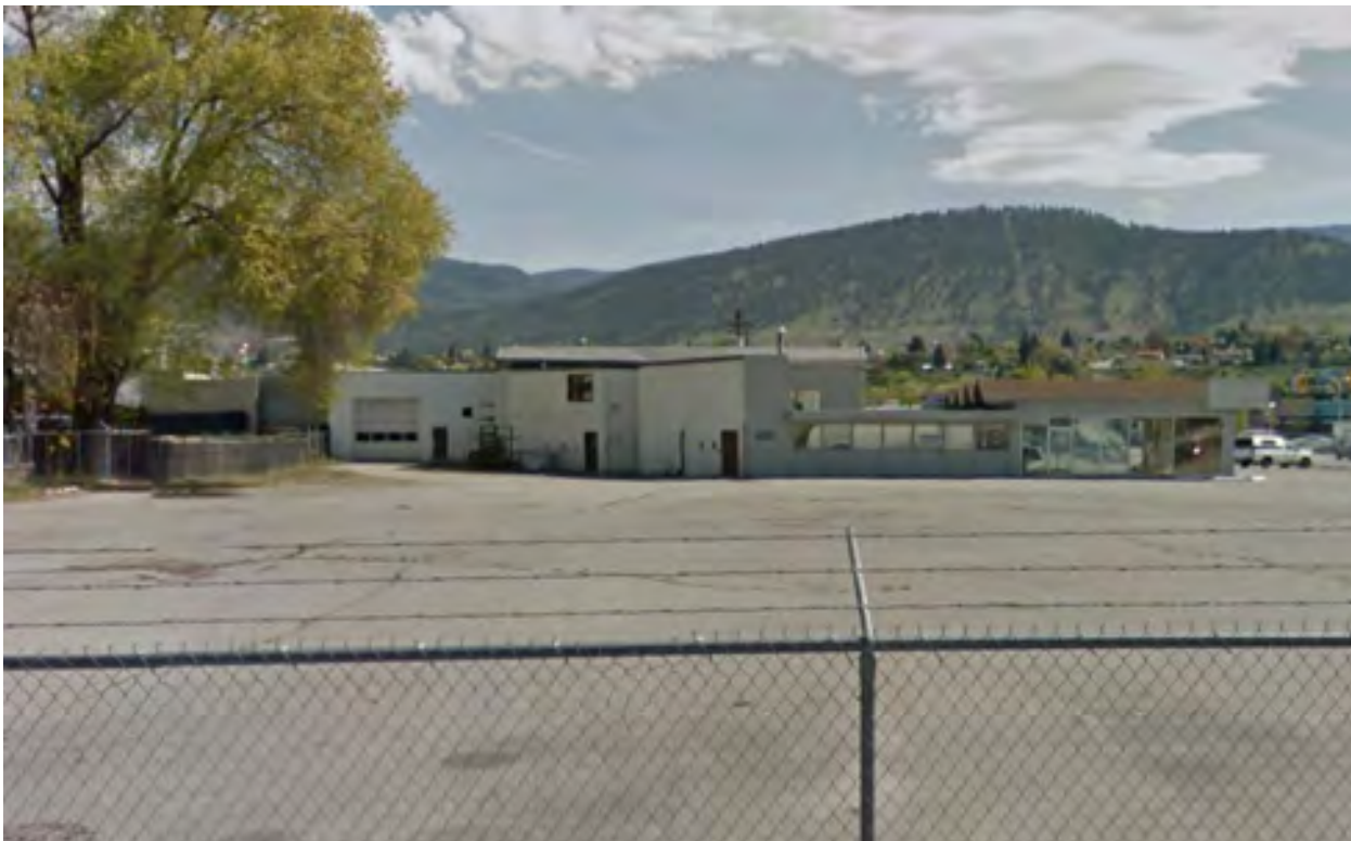
Image of subject property from Brunswick Street looking east, with the main building and detail shop in the mid ground
