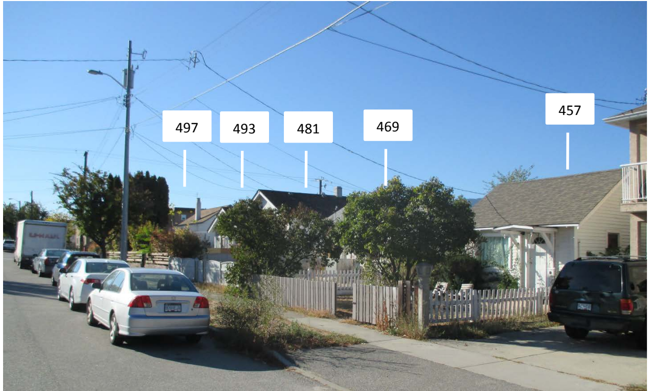
Figure 3: View of properties to be demolished, Braid Street looking south
