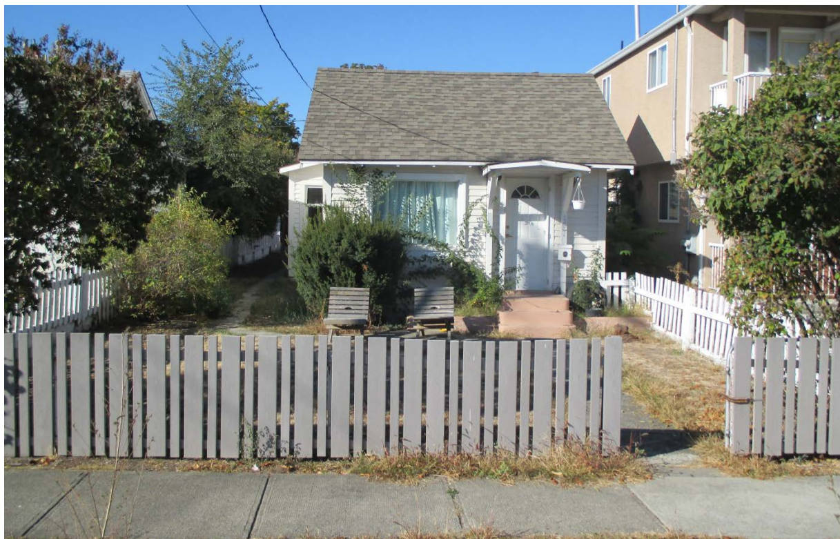
Figure 4: 457 Braid Street looking west. This home typical of homes being removed
