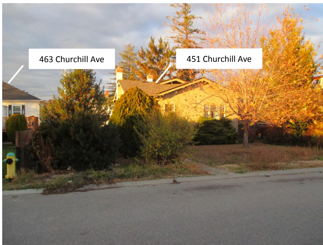
Figure 4: Looking toward the front of 451 Churchill Ave from Churchill Ave
