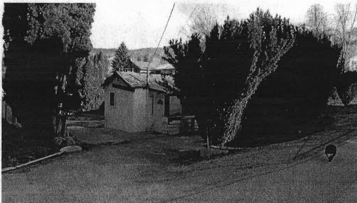
Figure 5: View from Cambie Place
