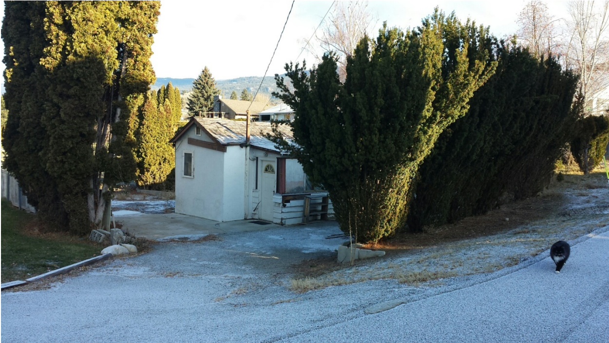
Figure 5: View from Cambie Place
