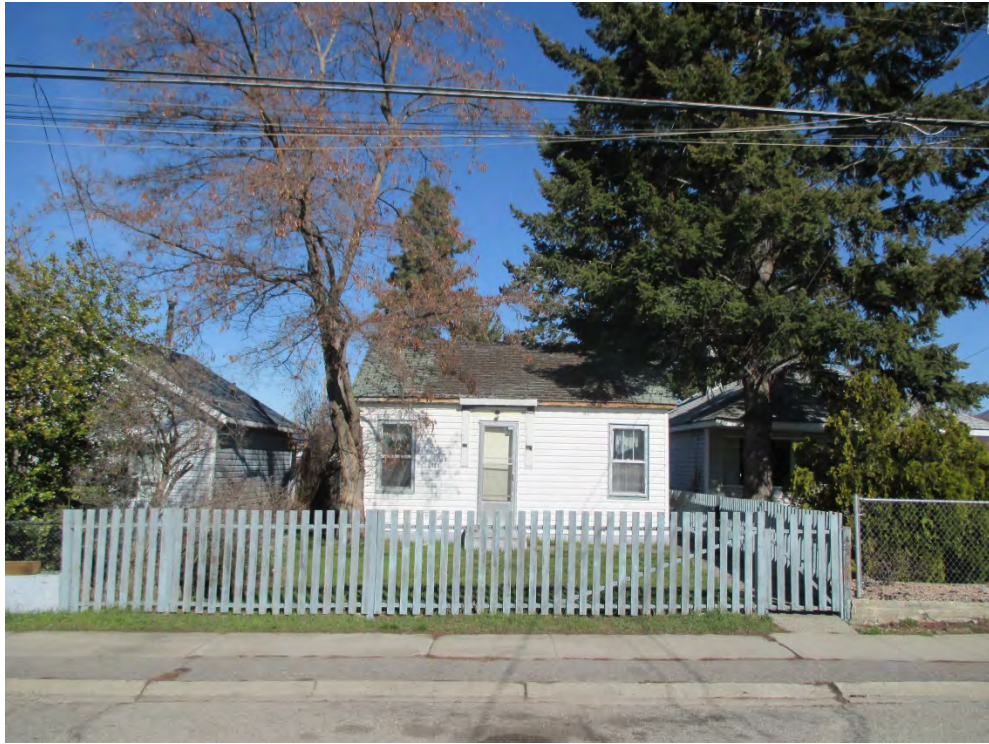
Figure 4: Looking north at 481 Nelson Avenue
