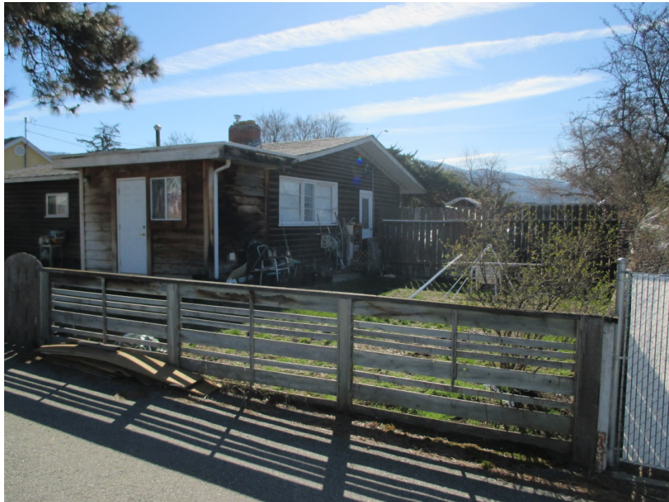
Figure 5: Looking south from alley at home to be removed
