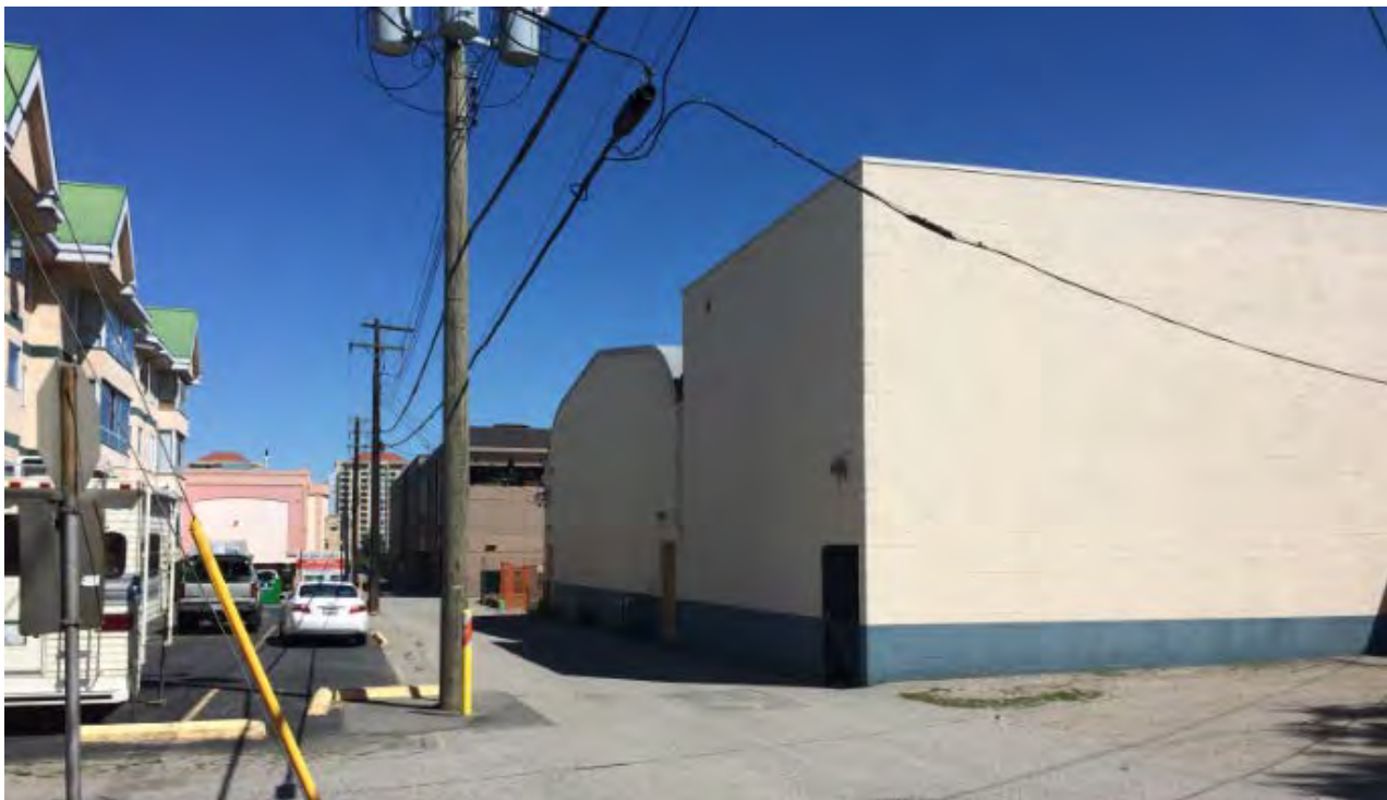
Figure 4: Image of subject building from rear lane, looking north, showing proximity to apartment building
