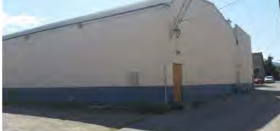
02 LOOKING EAST VIEW FROM ALLEY - EXISTING CONDITION (PHOTO)
