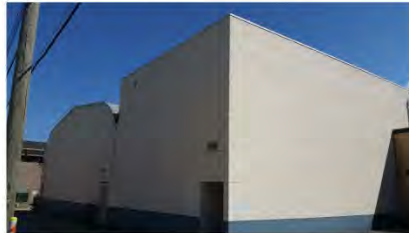
03 LOOKING NORTH VIEW FROM ALLEY - EXISTING CONDITION (PHOTO)
