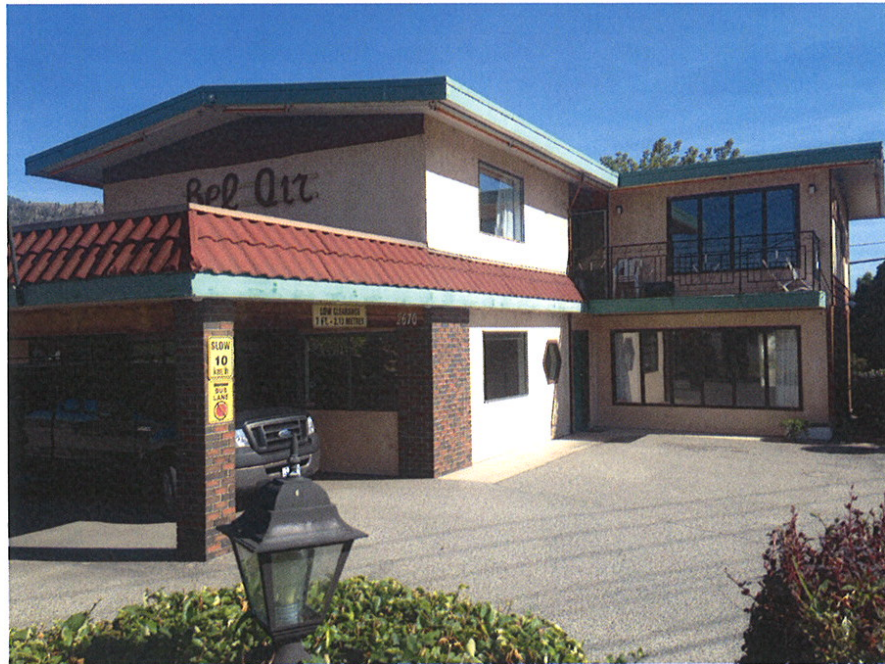
Figure 1: Former lobby and caretaker's suite
