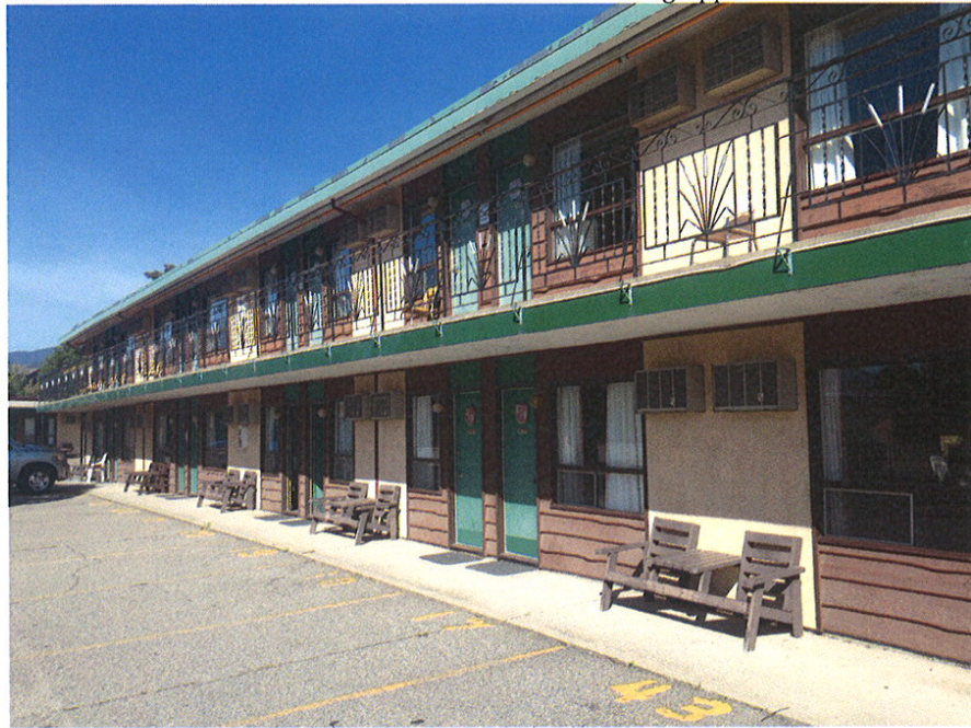
Figure 3: Close-up of east building, facade typical
