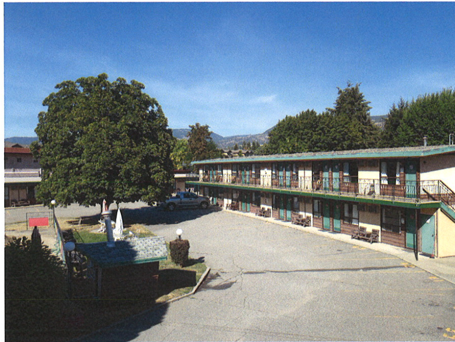
Figure 2: Inner courtyard area and two of three buildings
