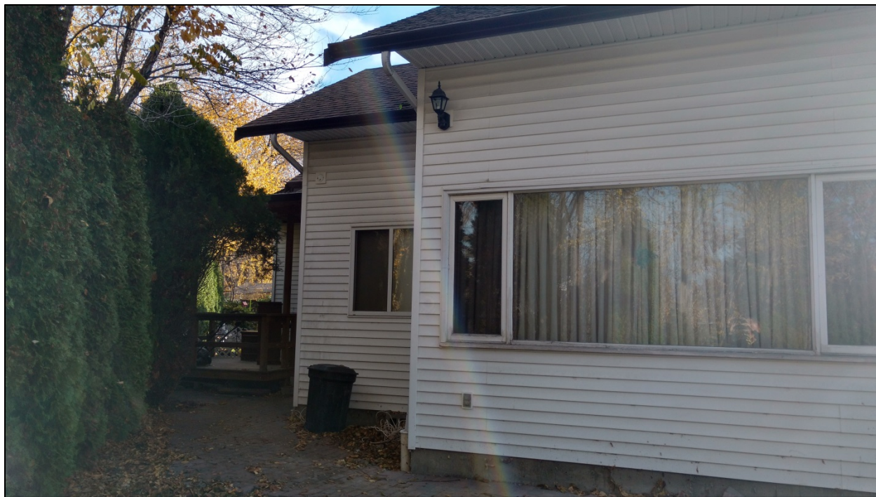
Figure 6: North East Side of building
