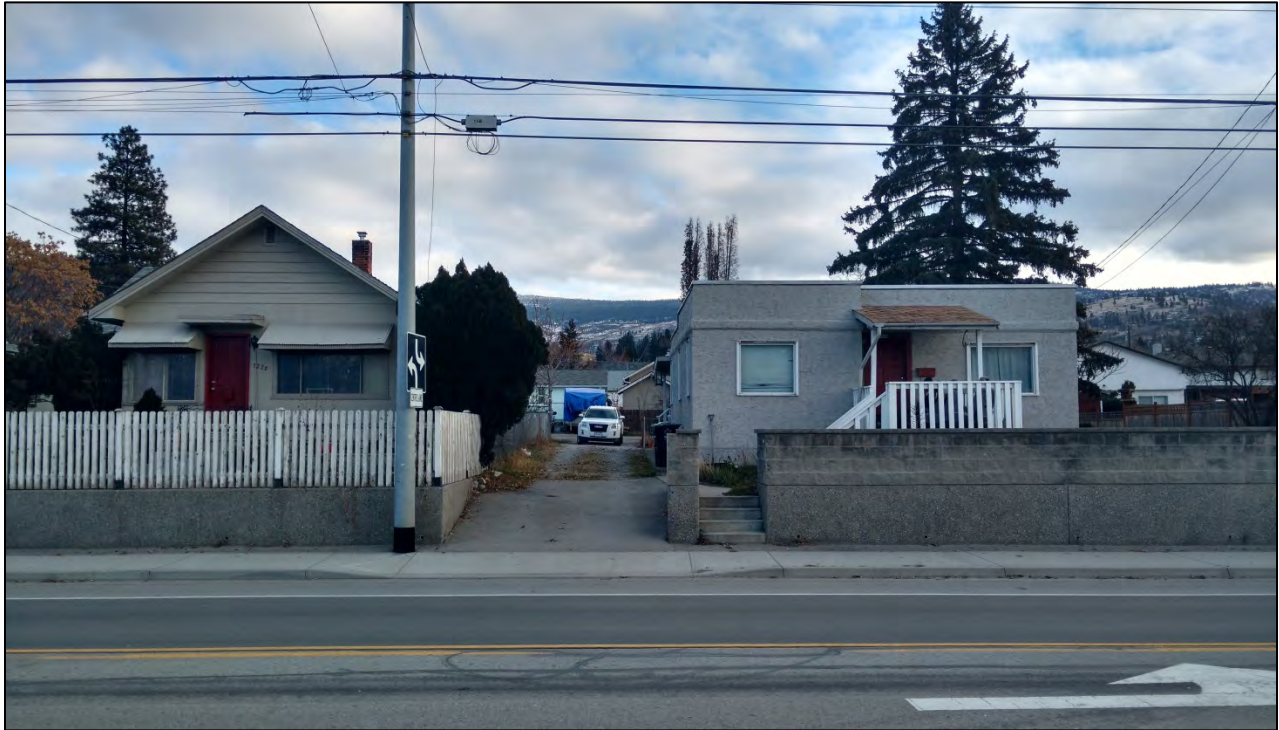
Figure 4: West View (from Government St.) showing existing Residents
