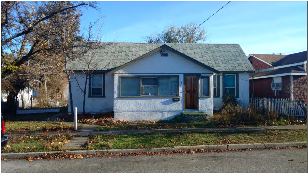
Figure 4: Street View of Subject Property (Existing House to be demolished)
