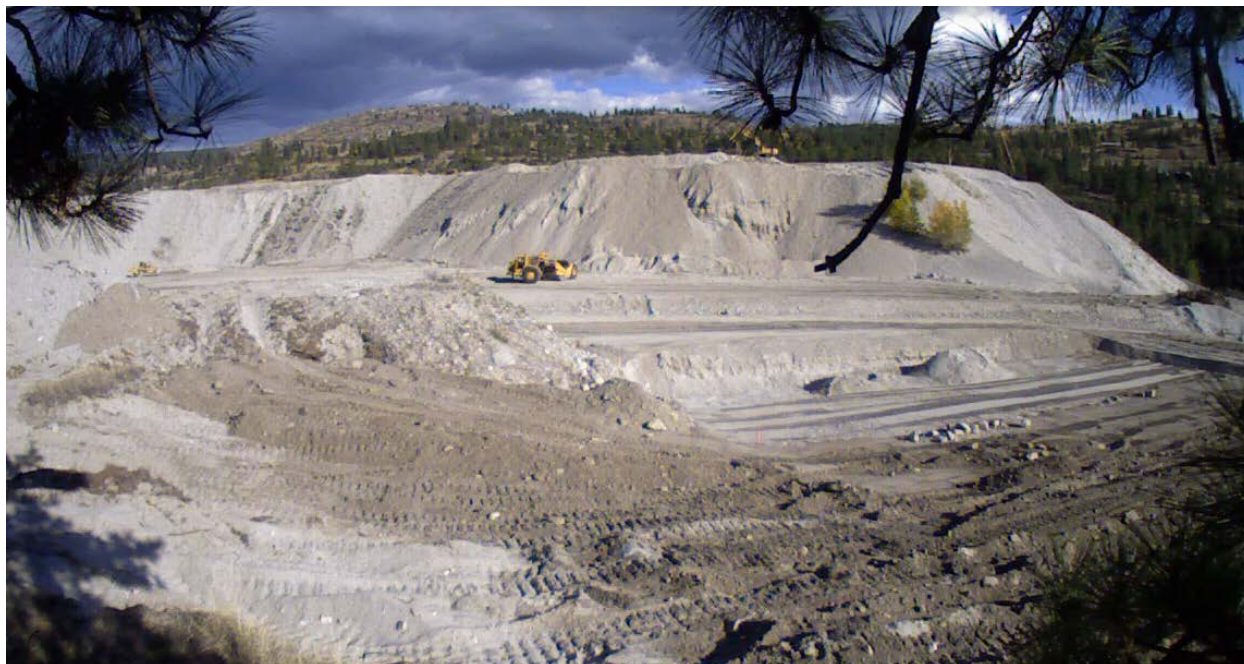
Figure 3: Image of subject lands looking east
