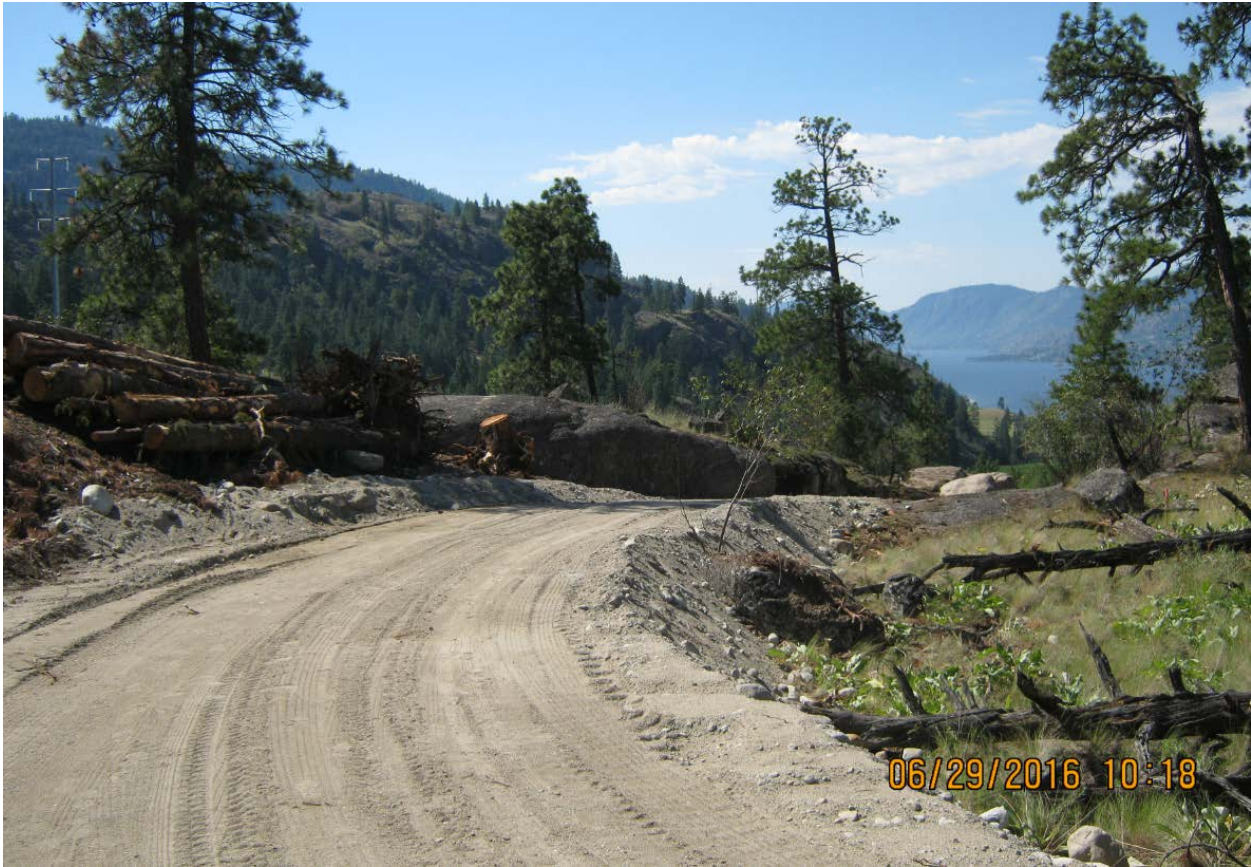
Figure 5: Driveway leading to Proposed Lot B, through neighbouring property
