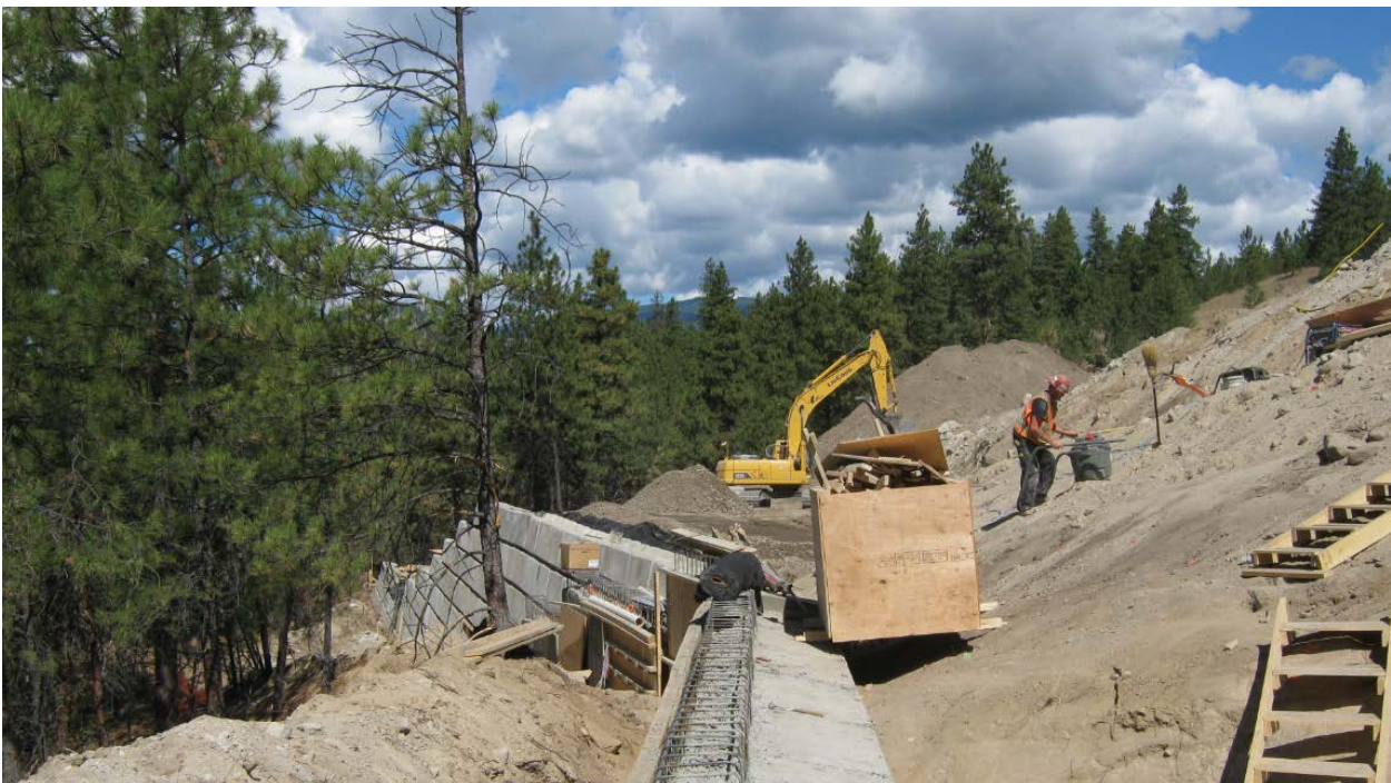
Figure 1: Image of cul-de-sac being roughed in, involving significant 'cutting' into the hillside
