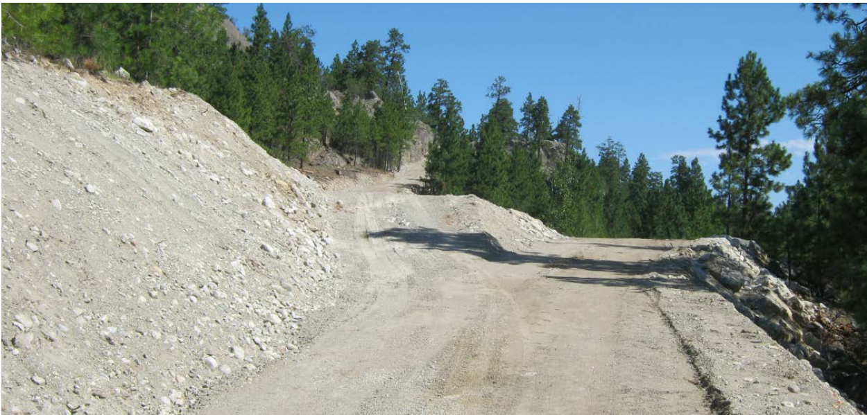
Figure 4: Split in driveway leading towards Proposed Lot B
