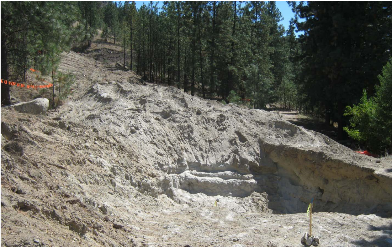
Figure 1: Image of cul-de-sac being roughed in, involving significant 'cutting' into the hillside
