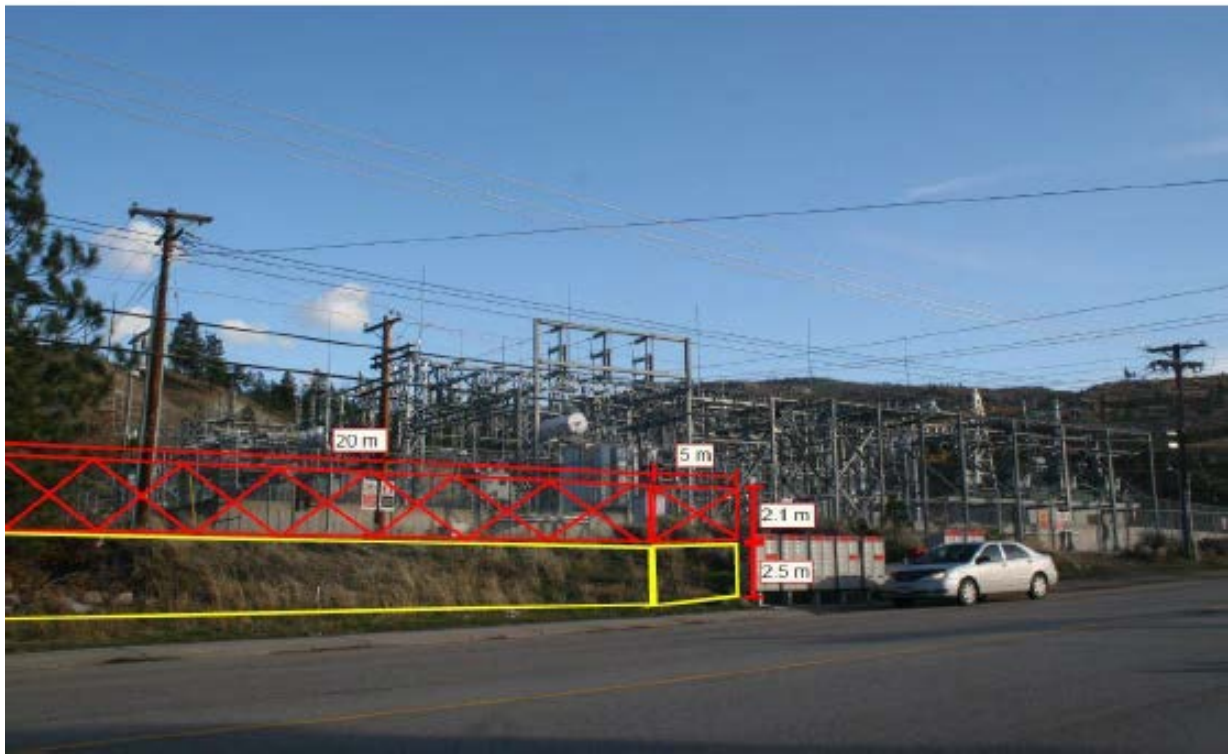
Figure 7: Proposed Fence & Retaining Wall along Carmi Avenue
