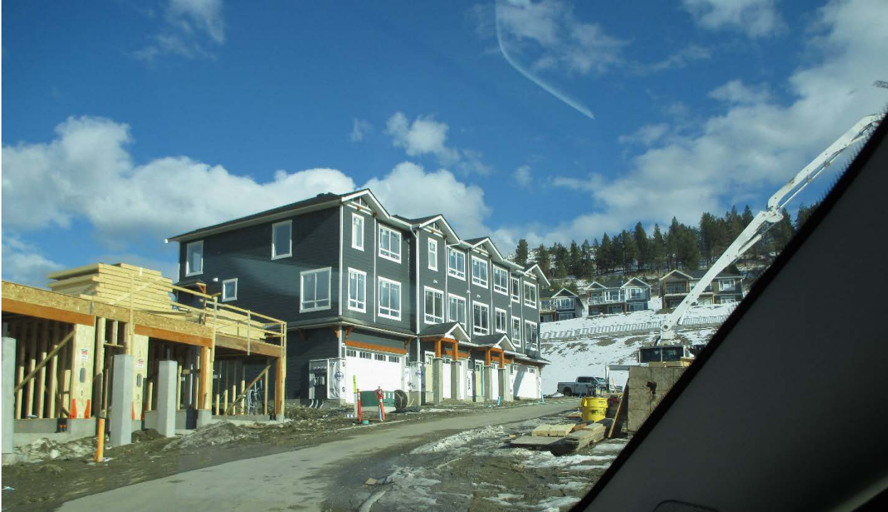
Figure 6: Townhouses currently under construction at Sendero Canyon
