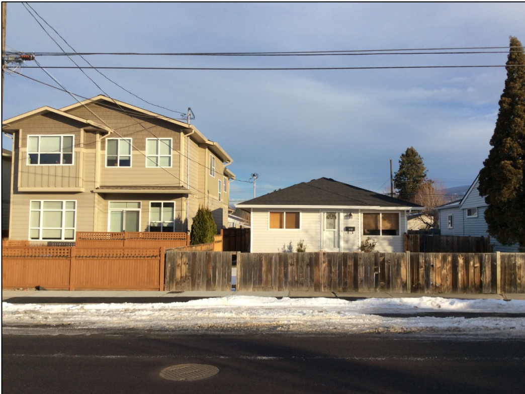
Figure 5: South View (from Douglas Avenue). Subject Property is on the right
