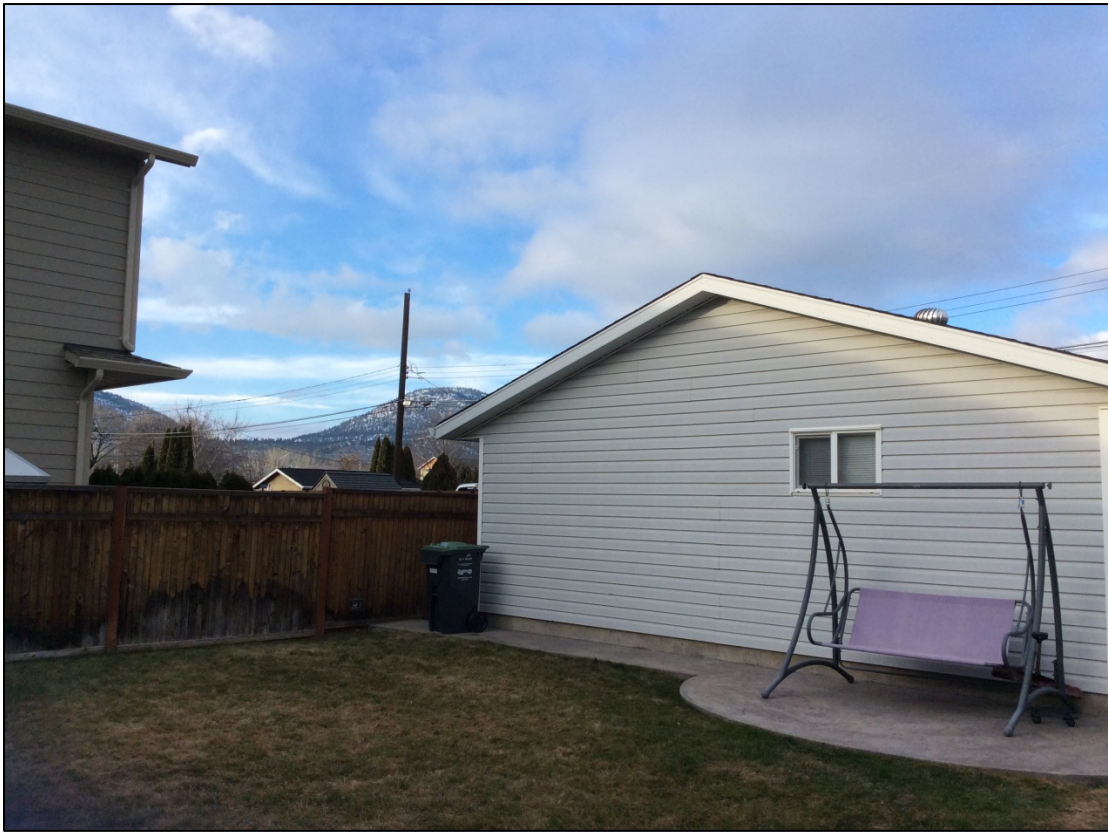
Figure 6 South View of Existing Garage
