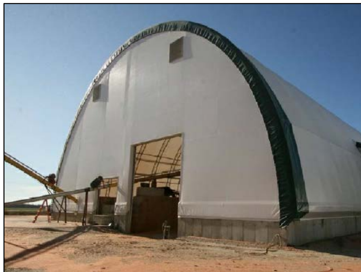
Figure 9: Similar Britespan Building
