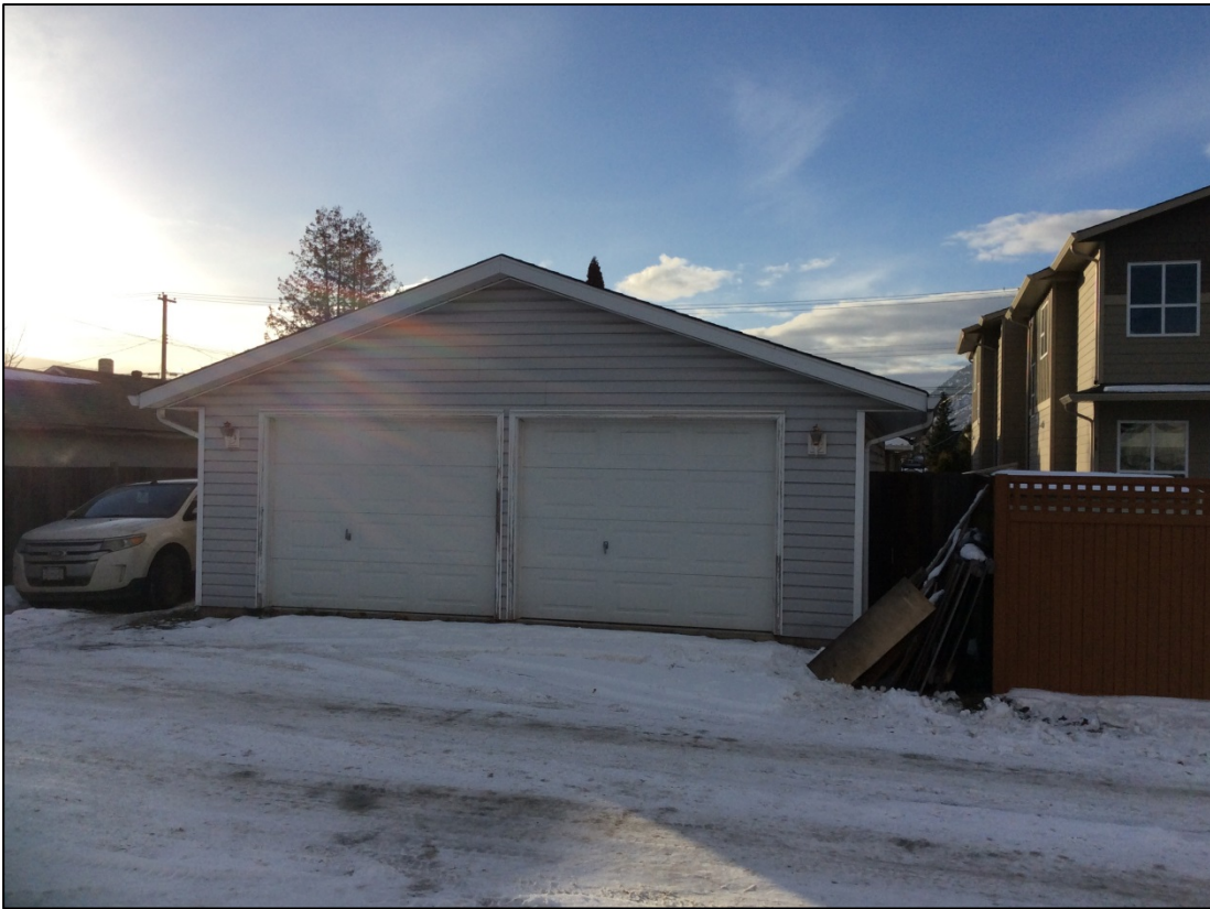
Figure 4 North View of Subject Property (from Lane)
